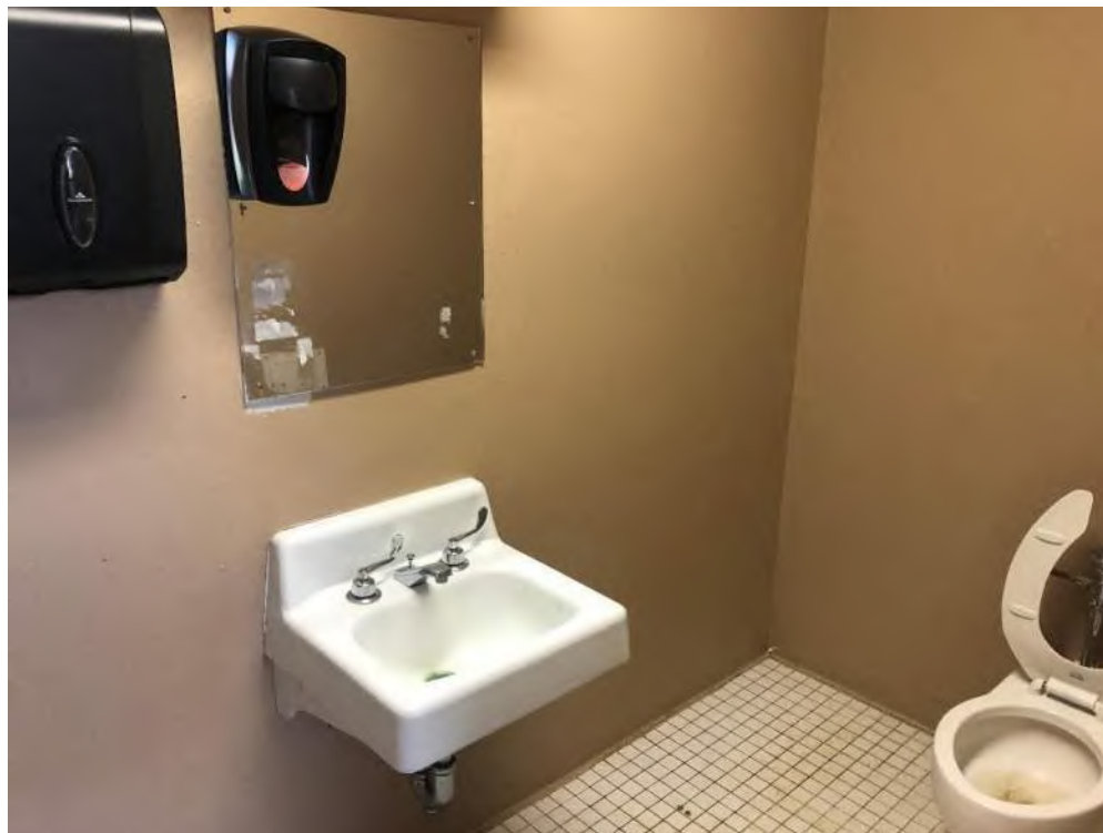
Photo 8: View of a typical white ceramic sink that has a lead coating.
