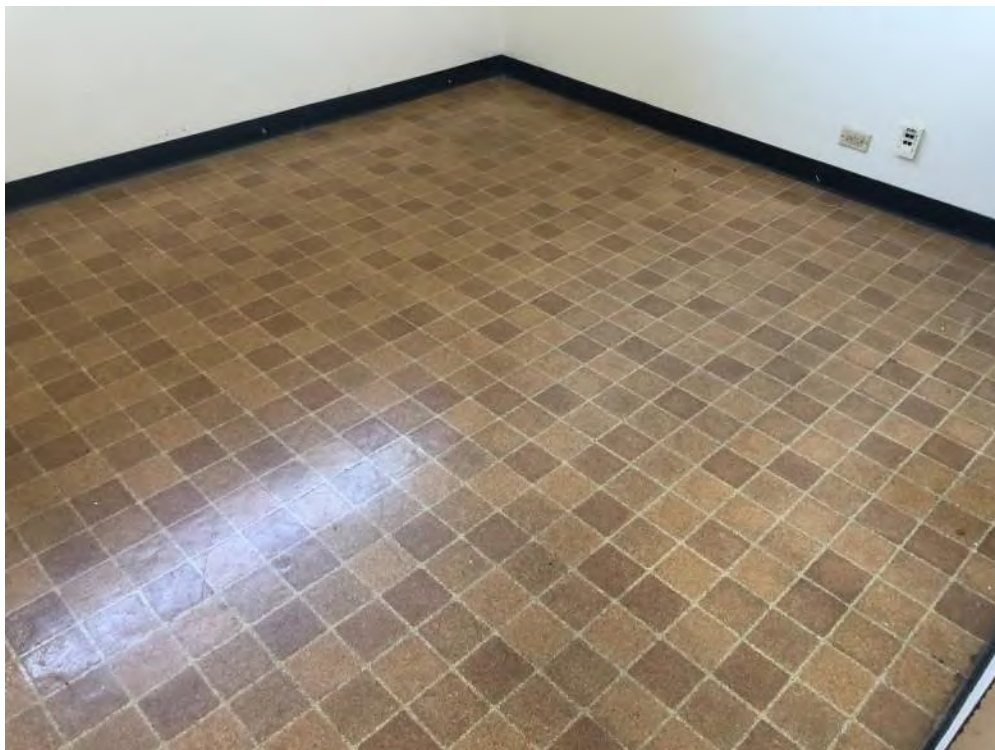
Photo 4: View of the asbestos-containing brick pattern floor covering.
