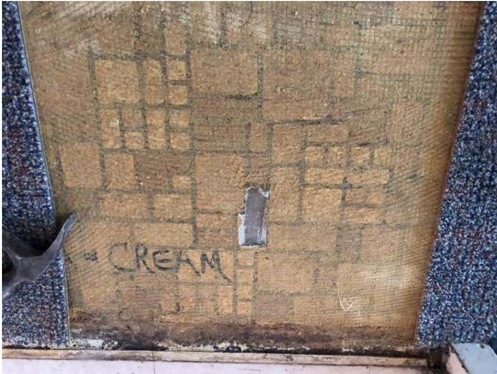
Photo 7: View of the asbestos-containing cream floor covering.
