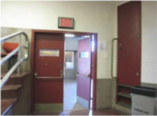
E-1 Entrance/Exit Door from inside Room 100. Requires Pull Station
