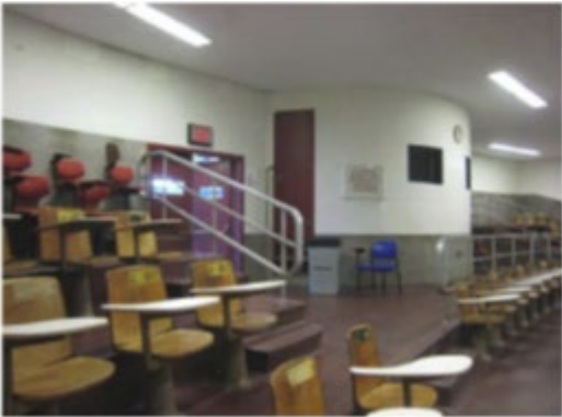
E-2 View of Projection Room. Exit Door requires Pull Station
