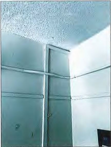
1 TYPICAL ELECTRICAL CONDUIT
