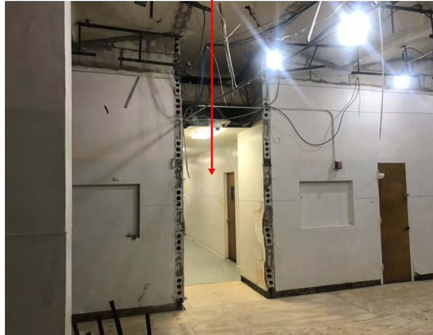
③d existing third floor room of Baker Building looking south
