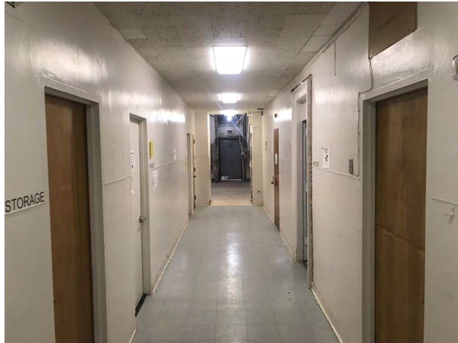
② third floor corridor of Baker Building approaching area of work
