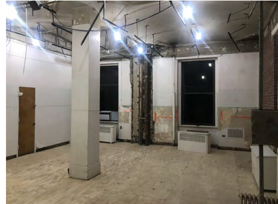
③e existing third floor room of Baker Building looking south and west
