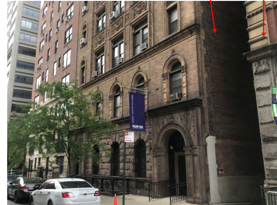
1c street level photos on East 67th Street looking west
