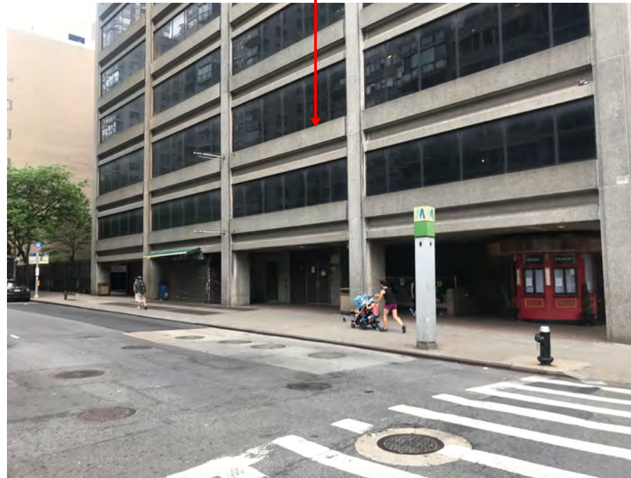
7a street level photo on East 68th Street between Lexington and Third Avenue looking southeast
