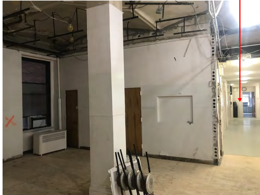
③c existing third floor room of Baker Building looking south and east
