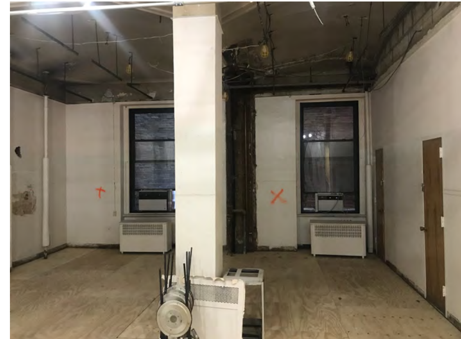
③b existing third floor room of Baker Building looking east
