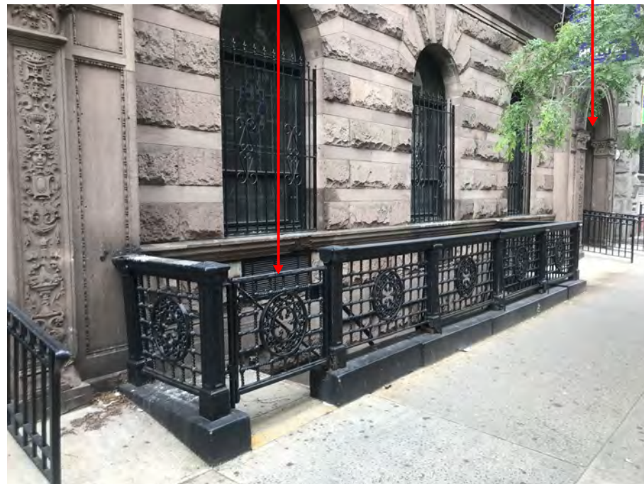
1d street level photo of stair to cellar entry
