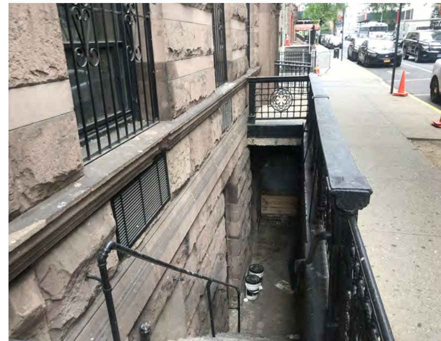
1e street level photo of stair to cellar entry looking down
