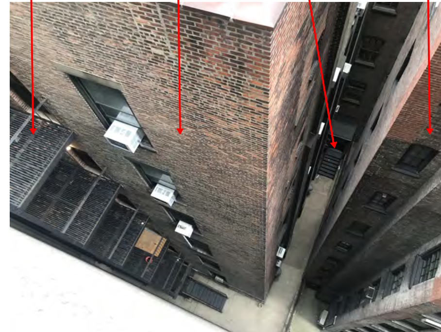
8b 8th floor terrace of East Building; photos looking down at area of work
