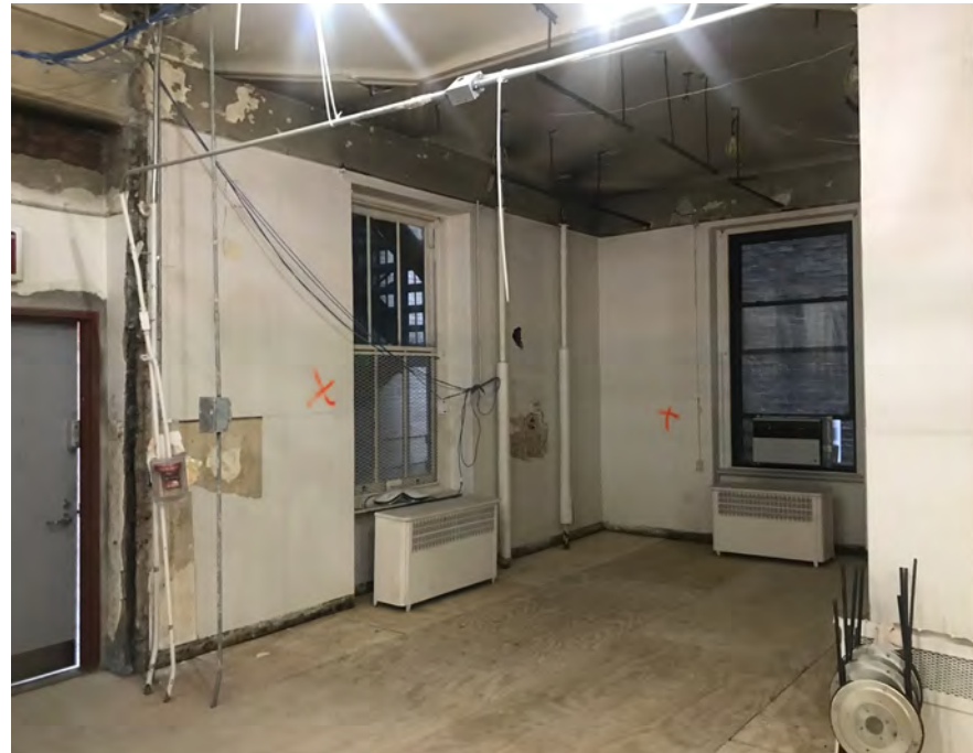
③a existing third floor room of Baker Building looking north and east
