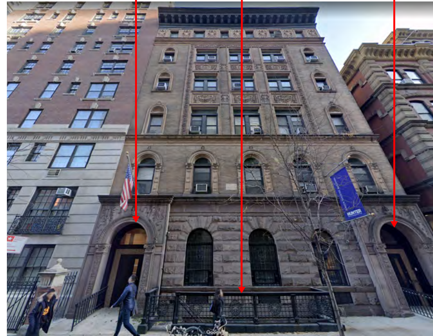
1b street level photos of building 1st floor entry and stairs to cellar
