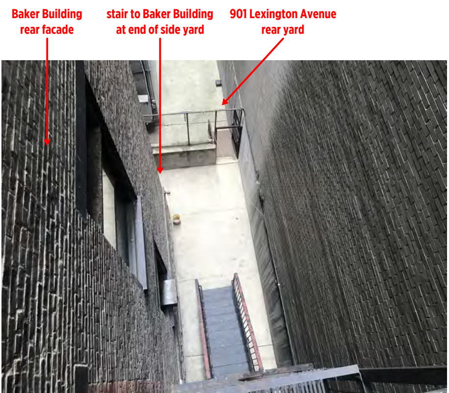
4d photos from third floor level on exterior stair looking down at rear yard ; northwest
