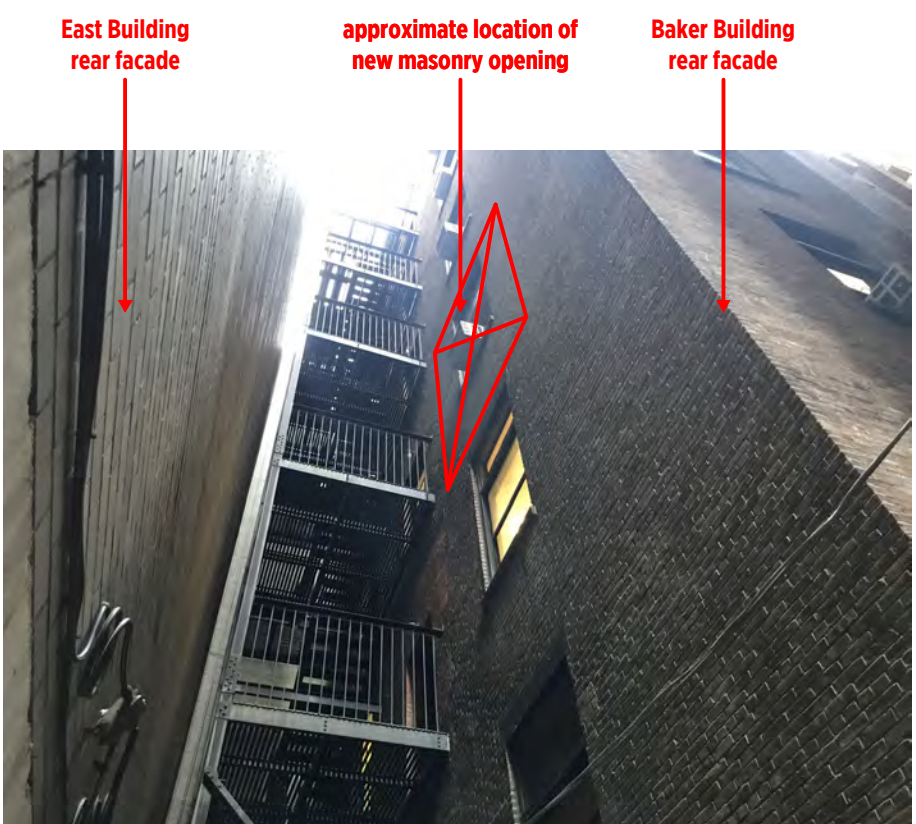
4g rear yard photos of exterior stair looking up south east
