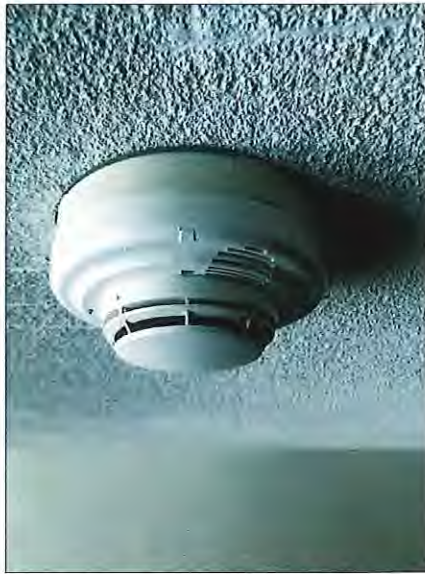
7 TYPICAL SMOKE DETECTOR
