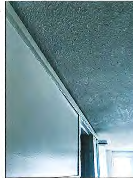
8 TYPICAL ELECTRICAL CONDUIT
