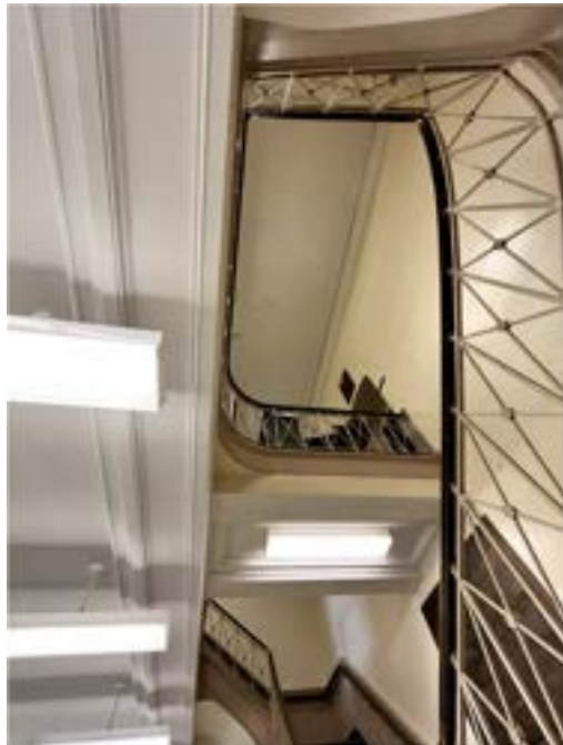
Photo 4: Two-Story Stair Opening
