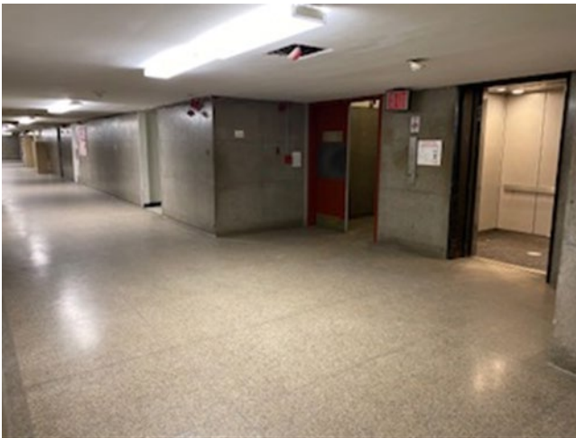
Photo 4: Basement level and view of corridor.
