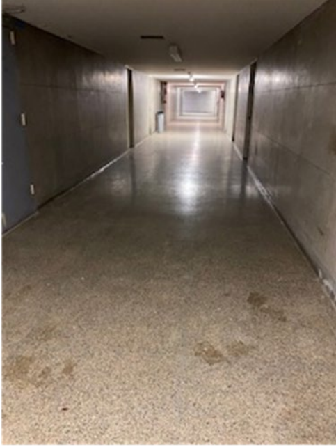
Photo 7: Corridor view at basement level.
