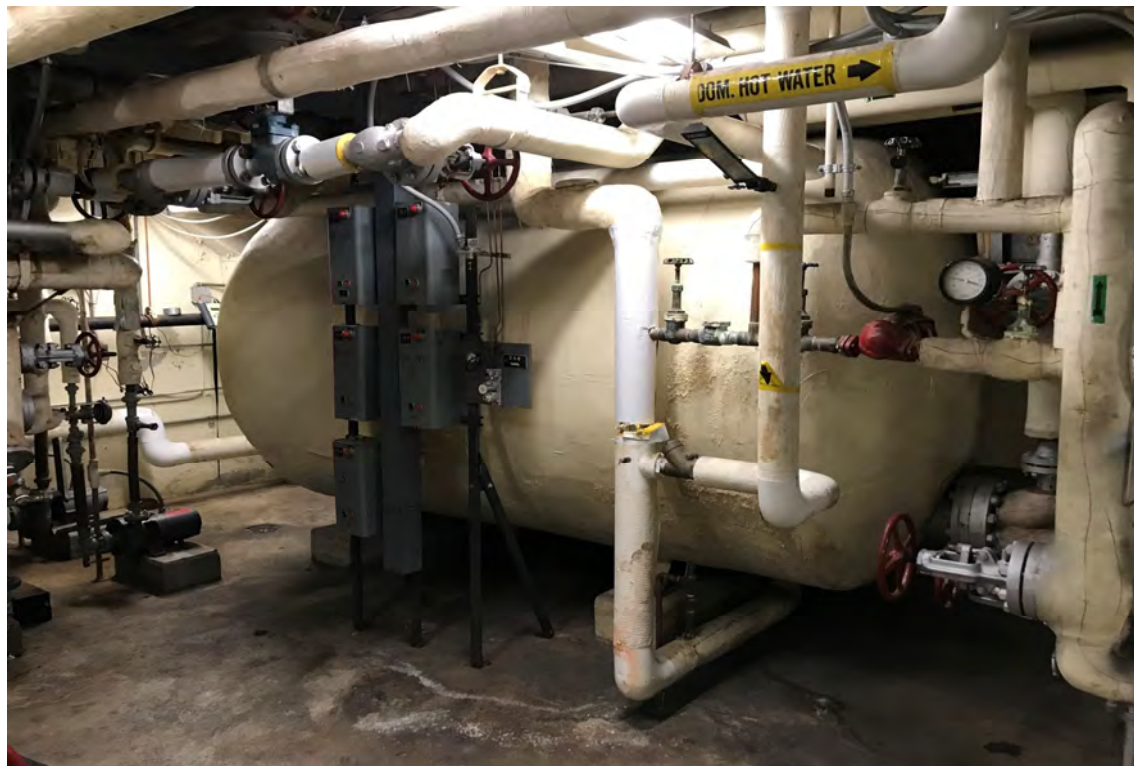
Hot water tank with asbestos-containing insulation in basement mechanical equipment room.
