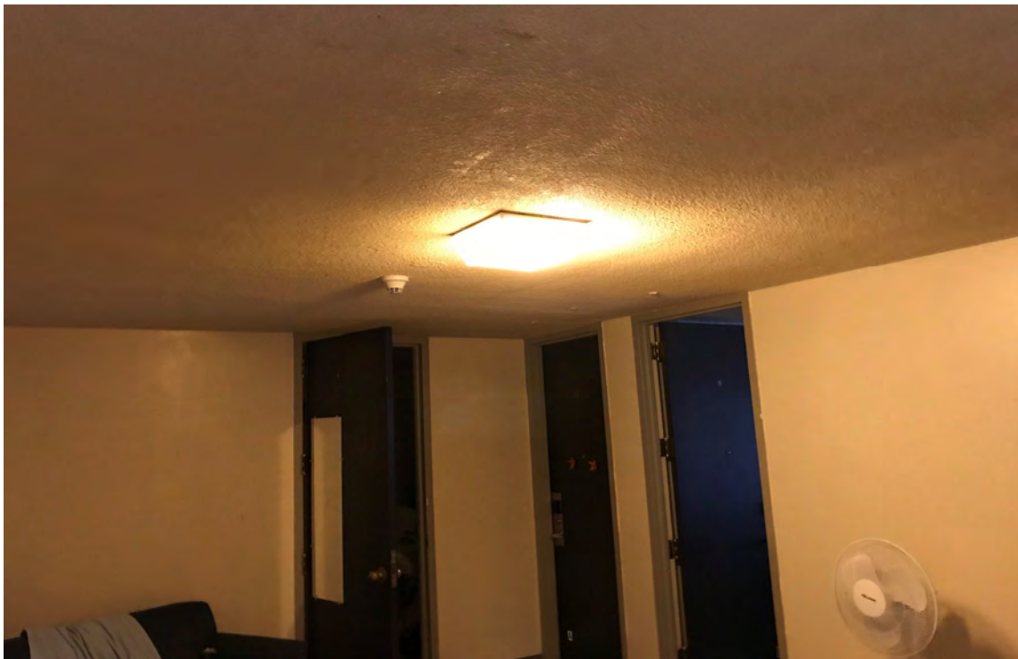
Asbestos-containing acoustical ceiling texture (ACT) in residential suites and stairwells throughout the building. Note typical light fixture with asbestos-containing wire insulation.
