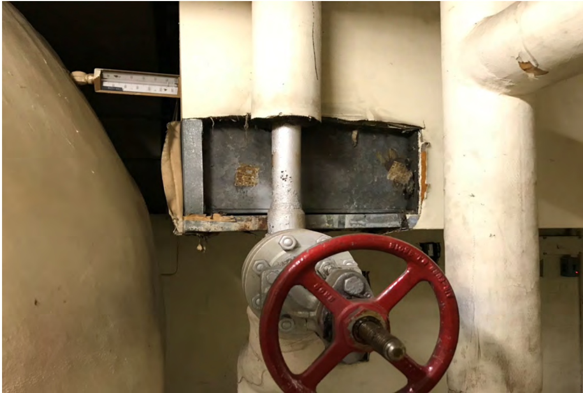
Asbestos-containing brown pin mastic for duct insulation in basement mechanical equipment room.
