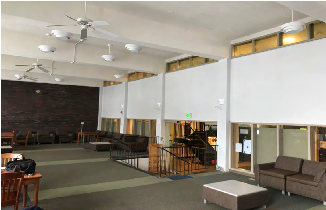
Clerestory and storefront windows in main floor lounge with asbestos and PCB-containing window glazing compound.
