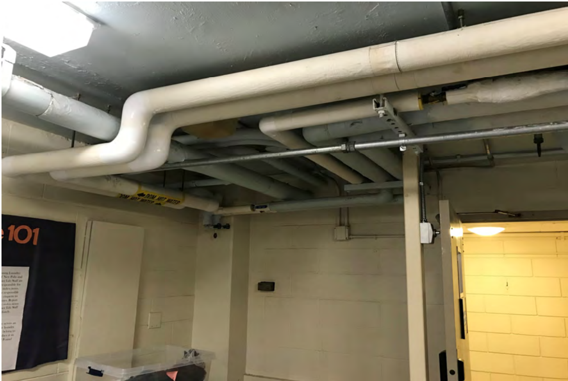
Piping with asbestos-containing mud pipe fitting insulation in basement laundry room (typical).
