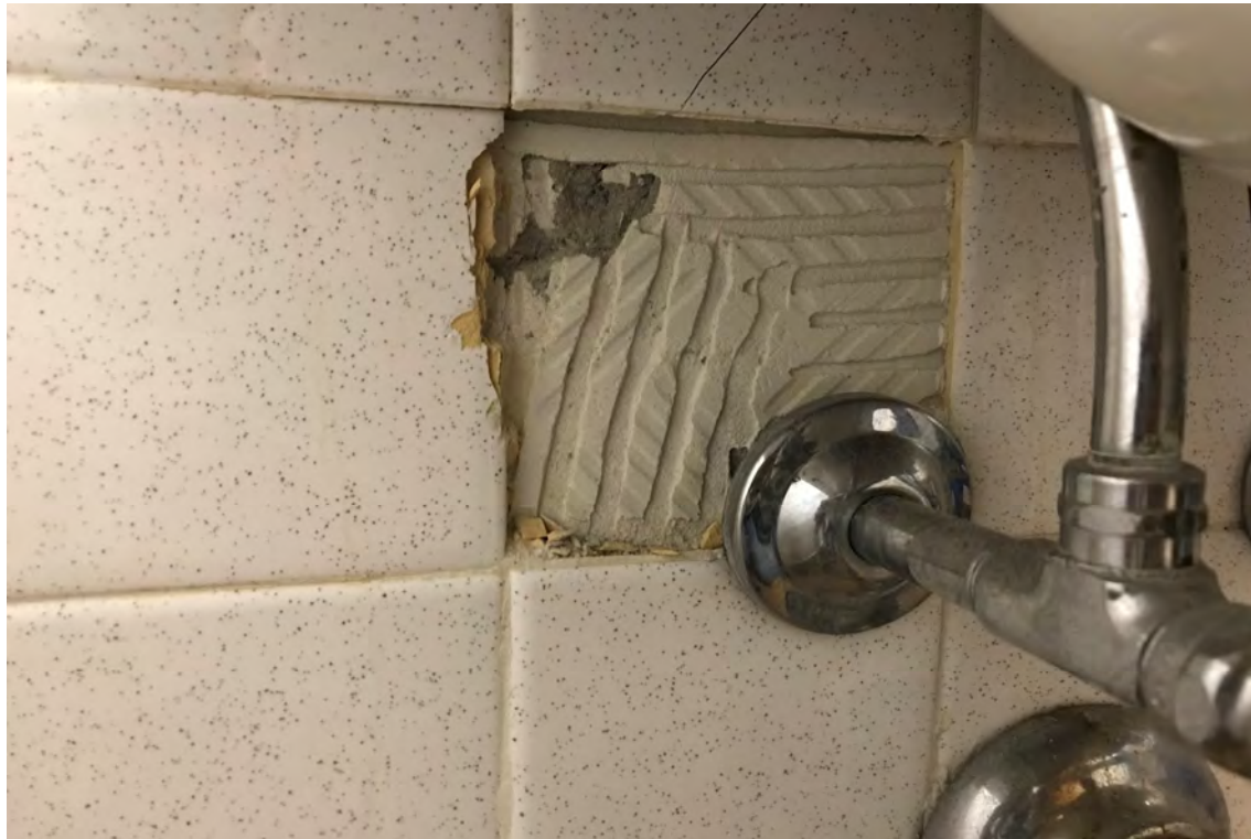
Thinset mortar for ceramic wall tile in bathrooms does not contain asbestos great than 1% and is considered a non-ACM.
