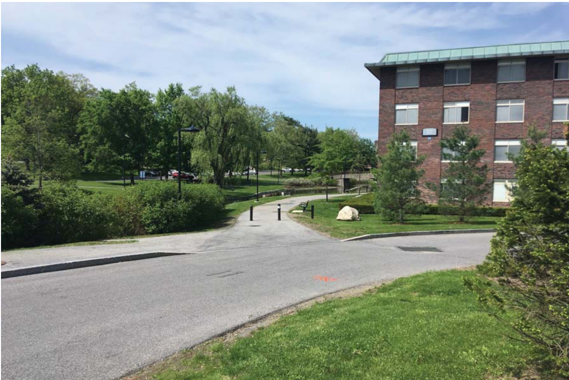
View north from the area of B-3
