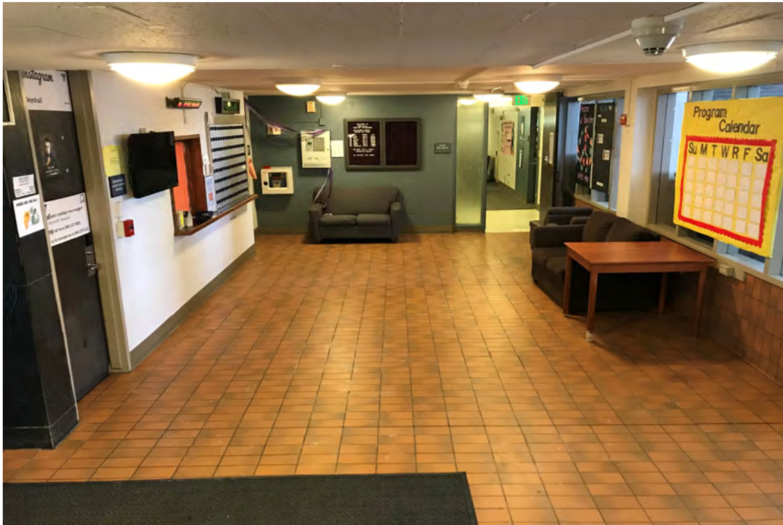
Control joint in lobby flooring with PCB-containing caulk.
