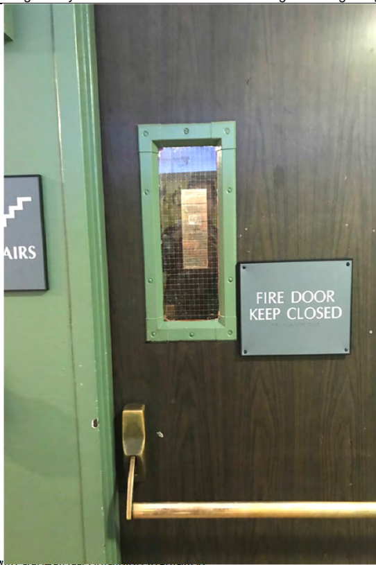
Typical stairwell fire door with asbestos-containing insulation.
