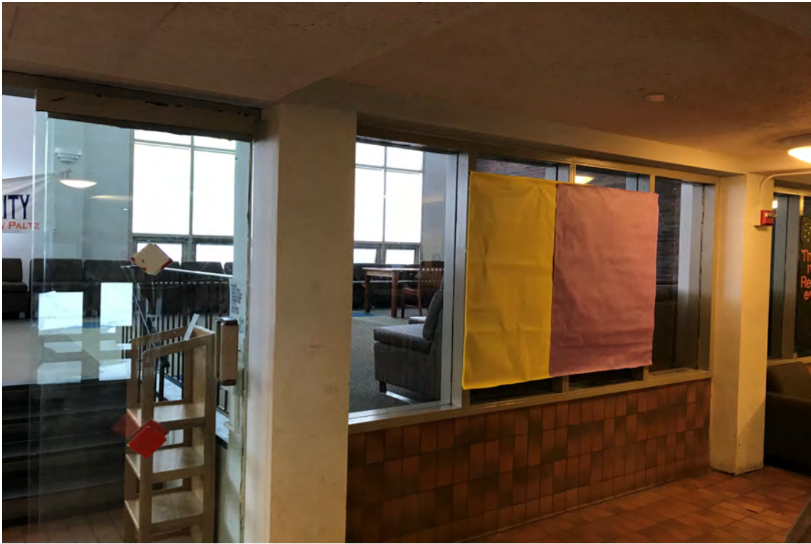
Interior windows between lounge lobby with PCB and asbestos-containing window glazing compound.
