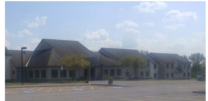
Figure 7-6. Mohawk Residence Hall
