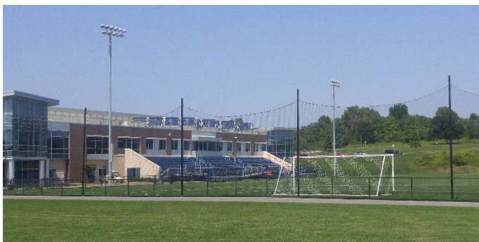
Figure 7-7. View of Wildcat Field House looking northeast; distant views of Proposed Project Site
