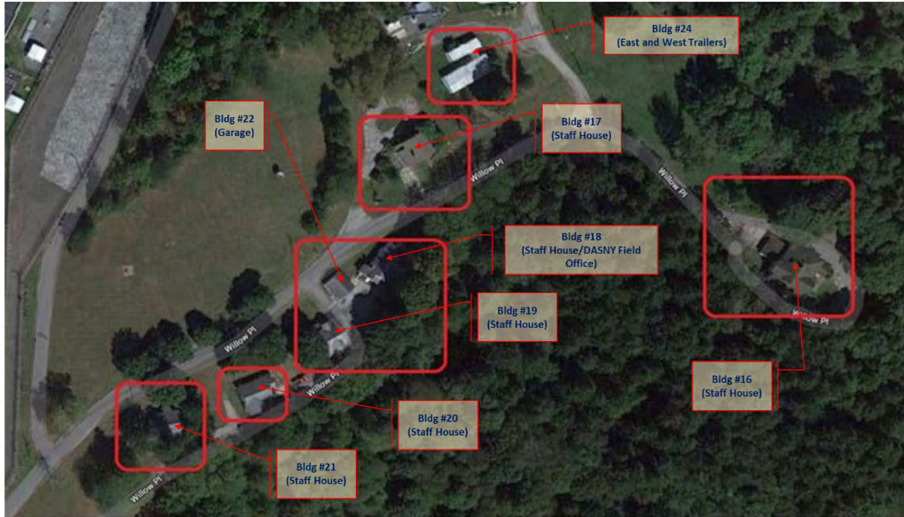
Figure 3. Staff Housing/Office Buildings to be Demolished
