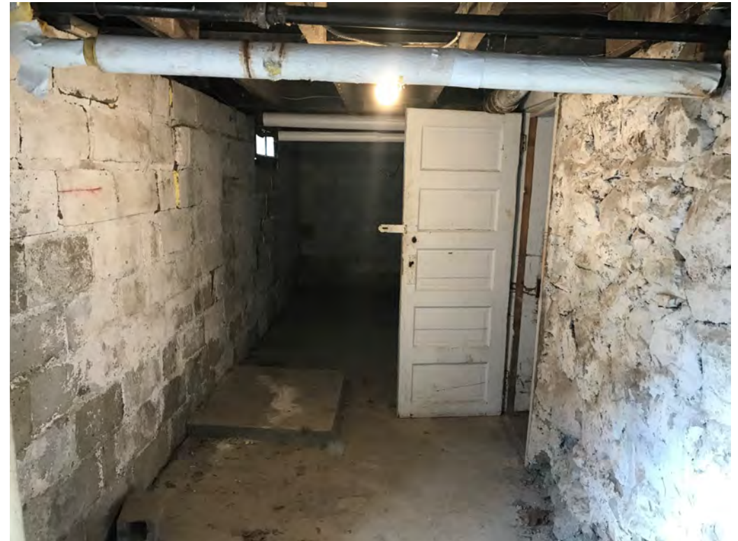
View of Basement East Room looking South
