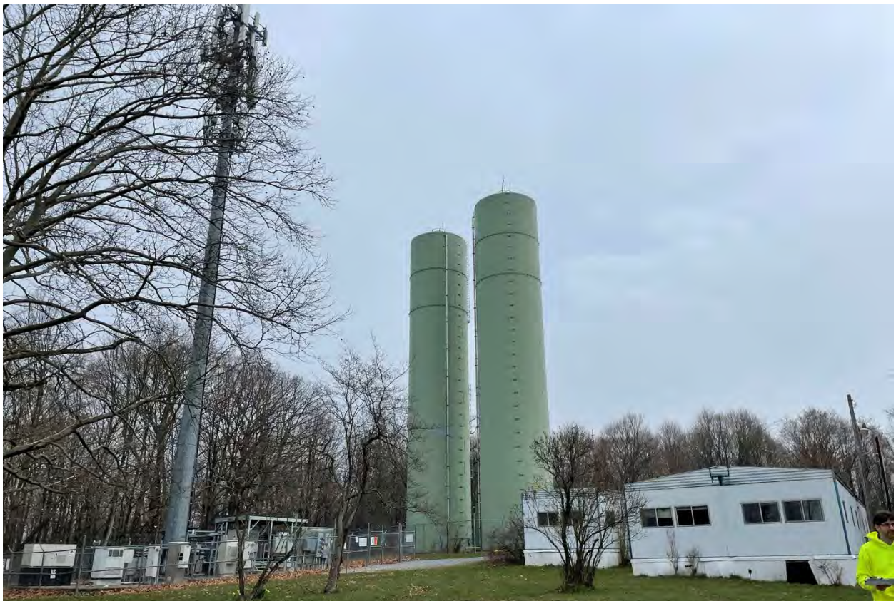
Photograph 18: Construction trailers (ca.1990), water towers, and telecommunications tower north of willow place, facing northeast from paved drive.
