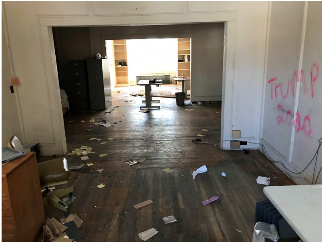
View of First Floor South Rooms looking East
