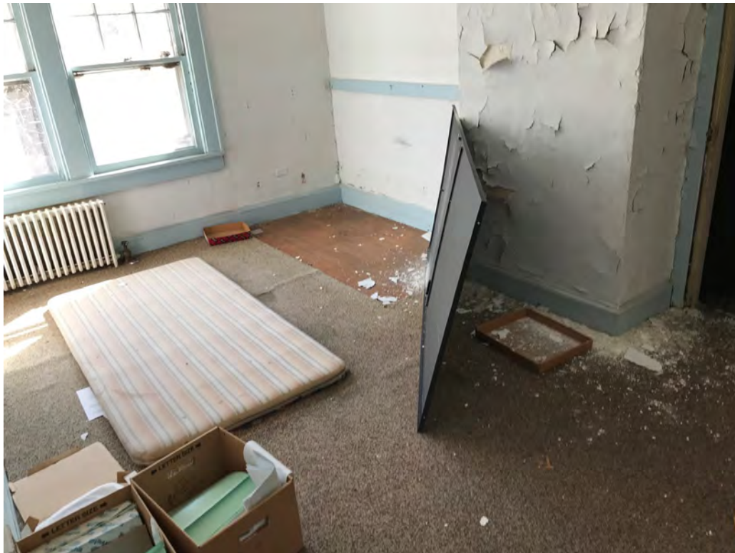
View of Second Floor Southeast Room looking Southeast
