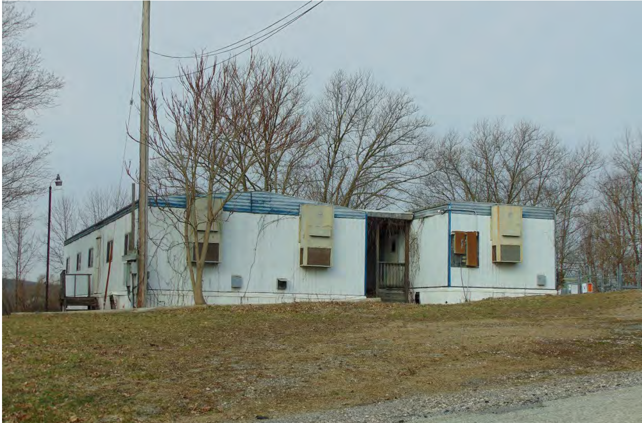
Photograph 15: East and west construction trailers installed on site after 1994, facing west to east elevations.
