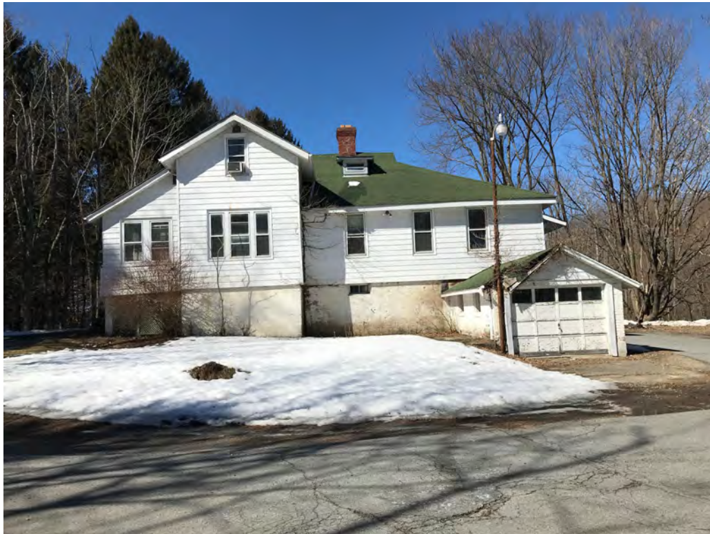
Exterior East Elevation
