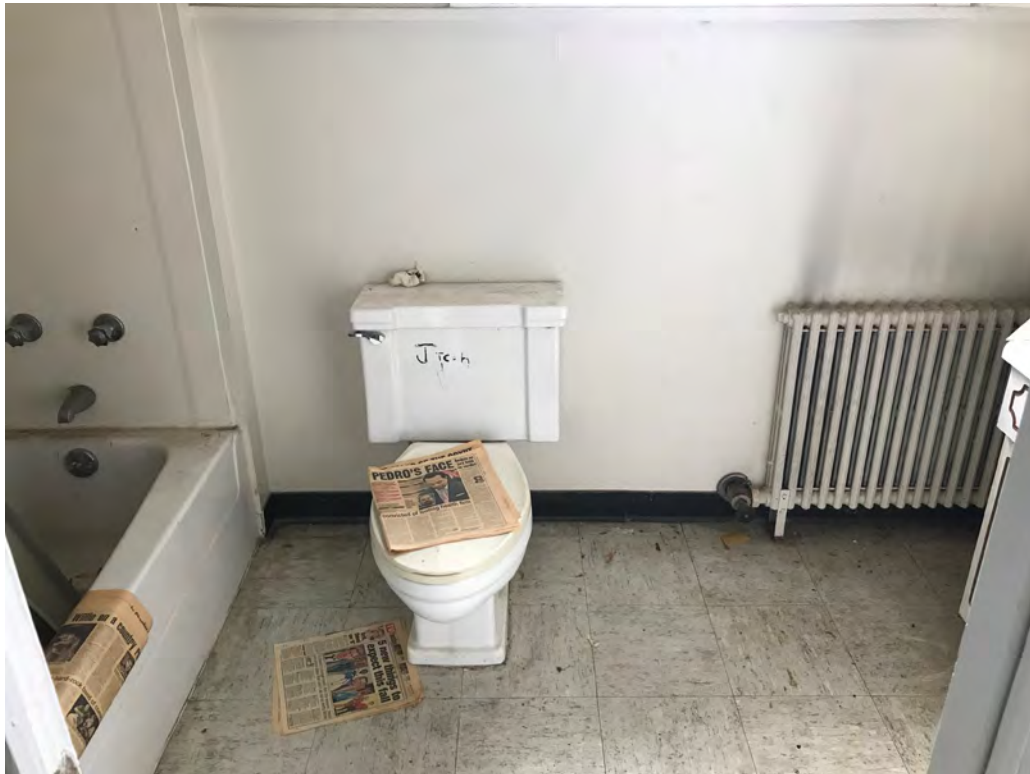
View of Second Floor Bathroom looking West
