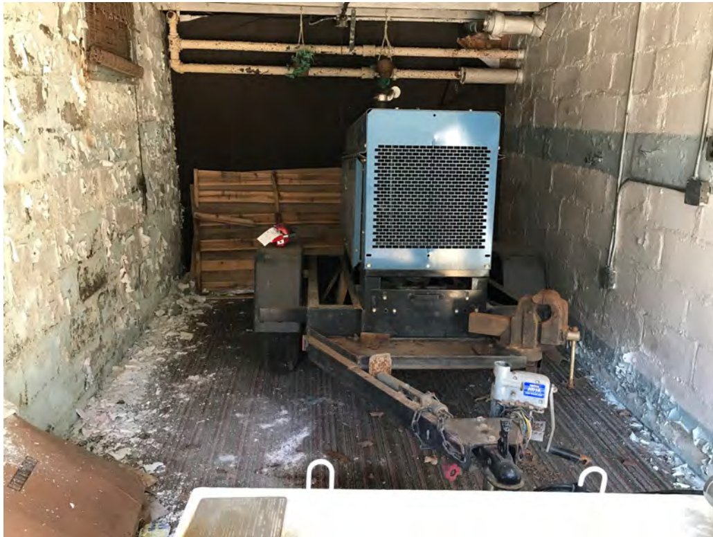
View of Basement Center Room (Garage) looking West
