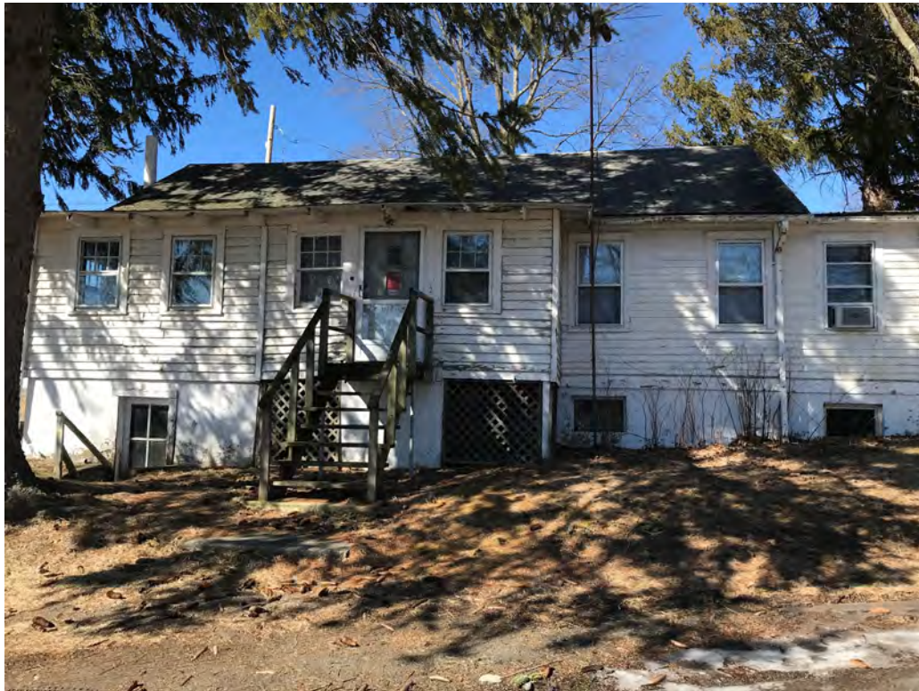
Exterior East Elevation
