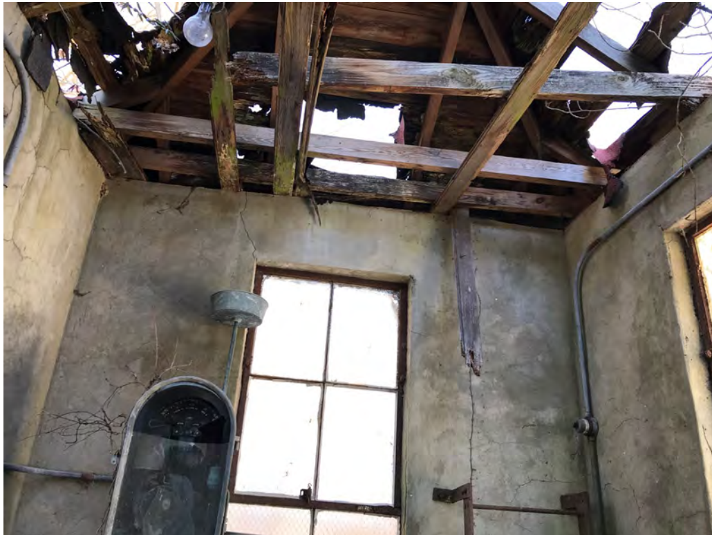
Interior Upper West Wall and Ceiling
