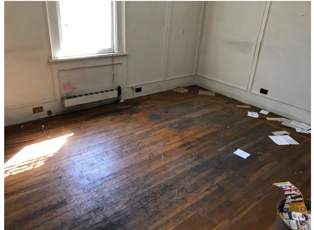
View of First Floor Southeast Office looking Southeast
