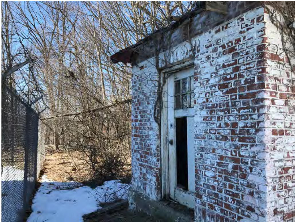
Exterior East Elevation
