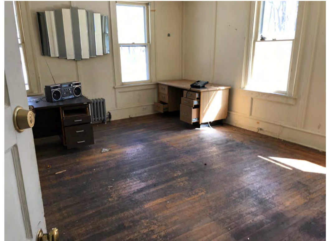
View of First Floor Northeast Office looking Northeast
