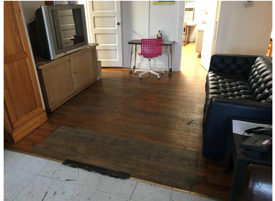
View of First Floor Center Room looking West
