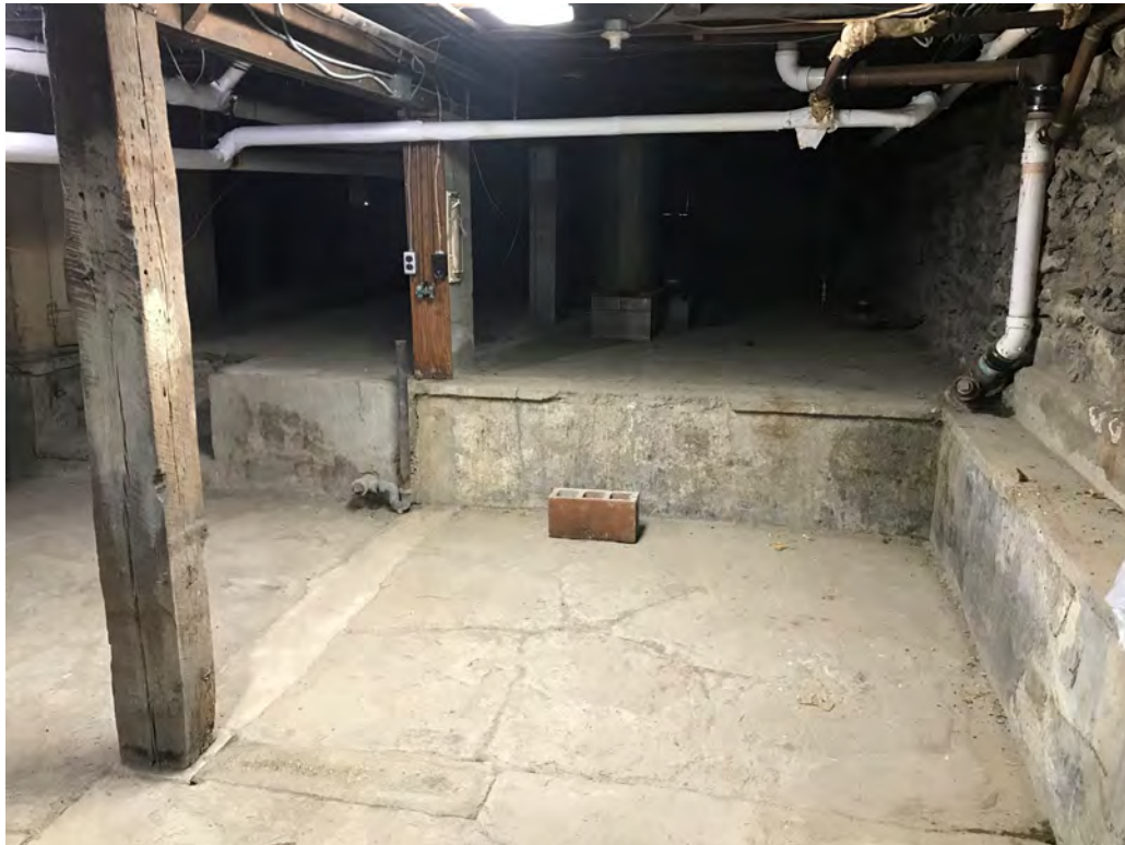
View of Basement Area looking South
