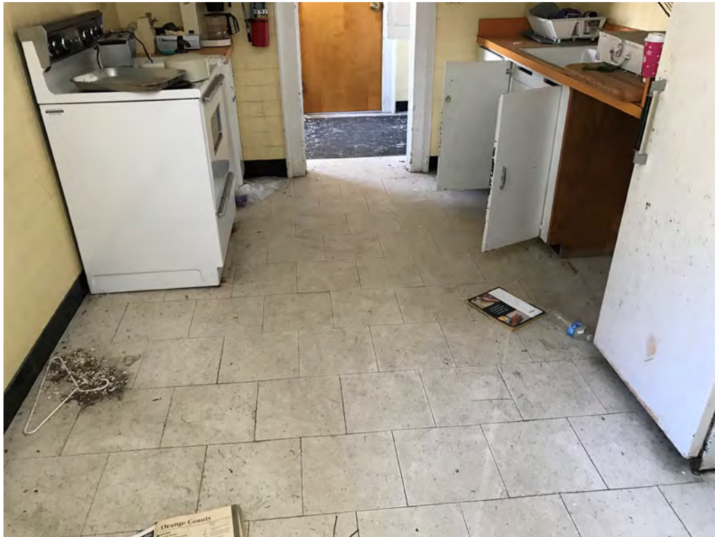
View of First Floor Kitchen looking North
