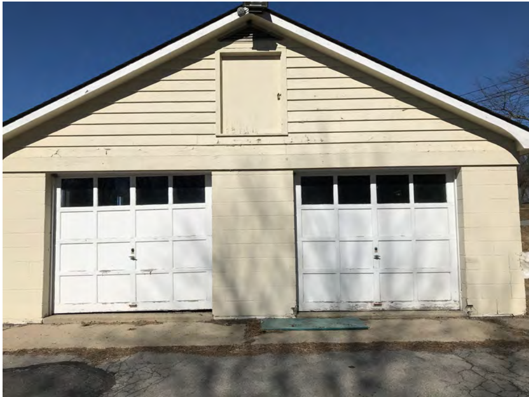
Exterior East Elevation
