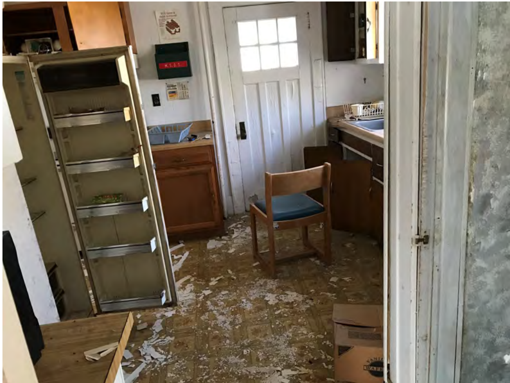
View of First Floor Kitchen looking West
