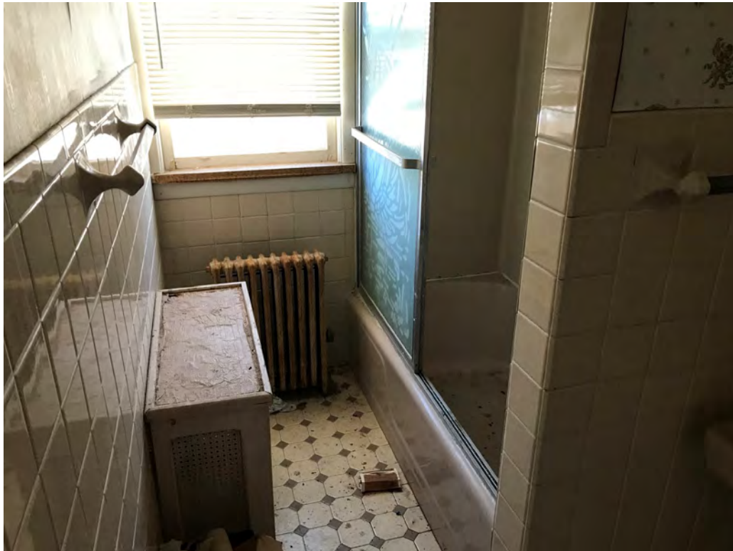
View of Second Floor Bathroom looking West
