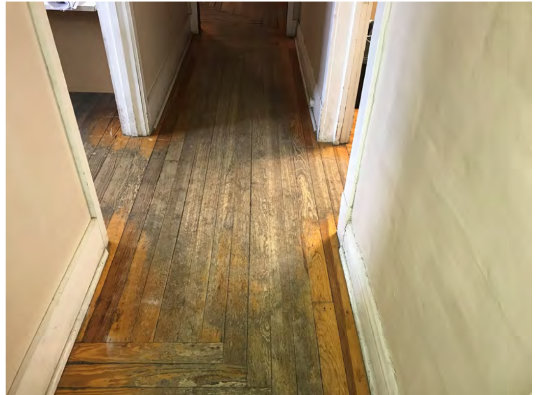
View of First Floor Corridor looking South
