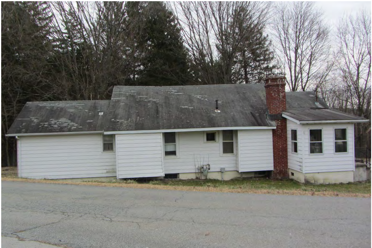
Photograph 6: Building 18 facing east to west elevation.
