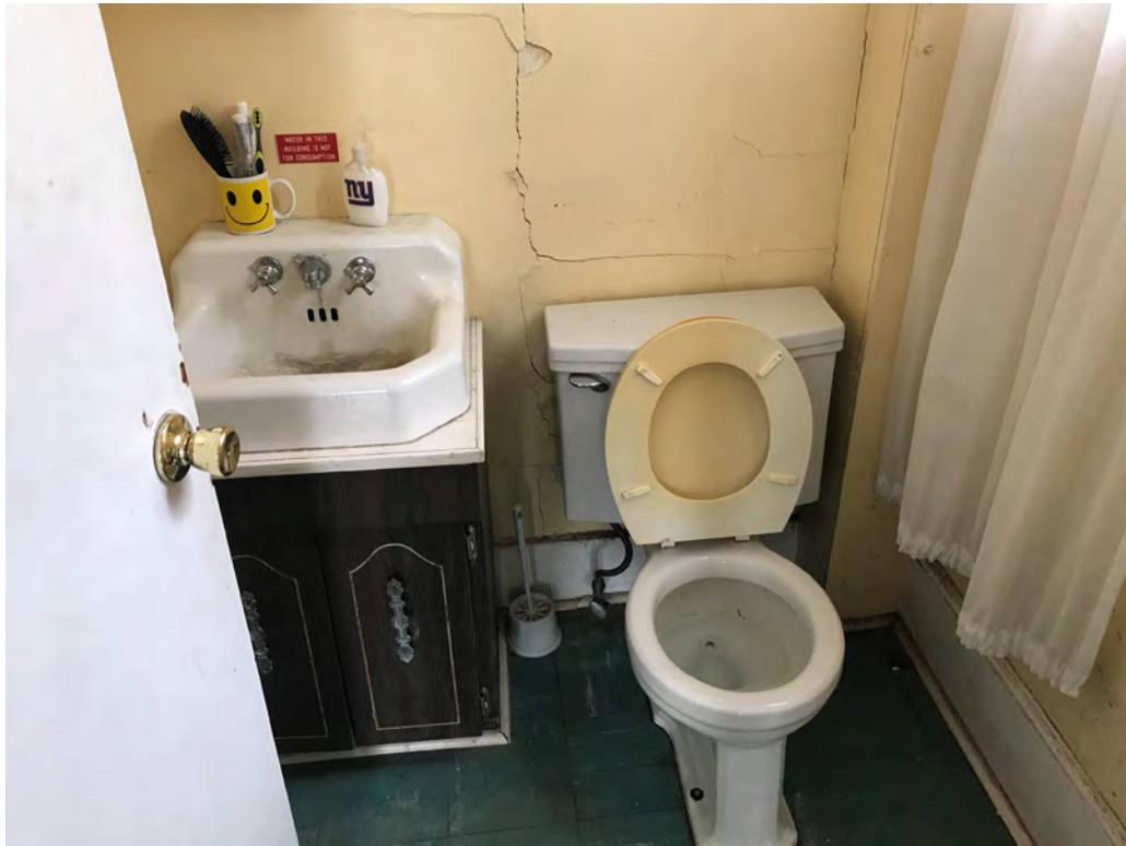
View of First Floor North Bathroom looking West
