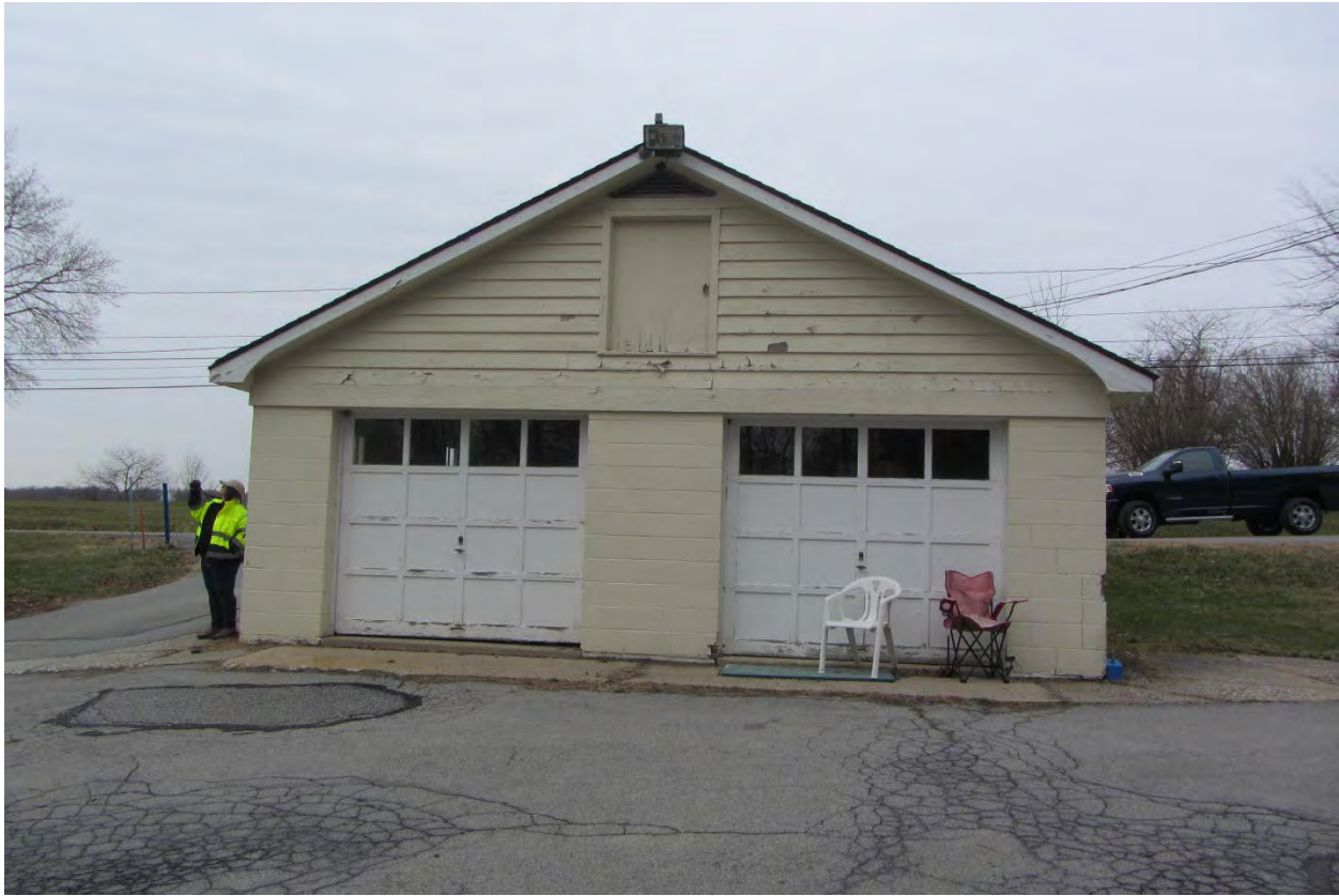
Photograph 13: Building 22 facing northwest to southeast elevation.
