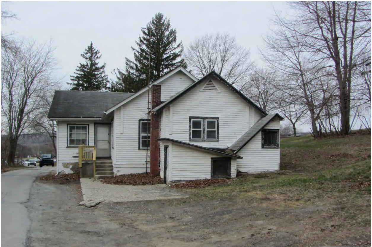
Photograph 10: Building 20 facing southwest to northeast elevation.
