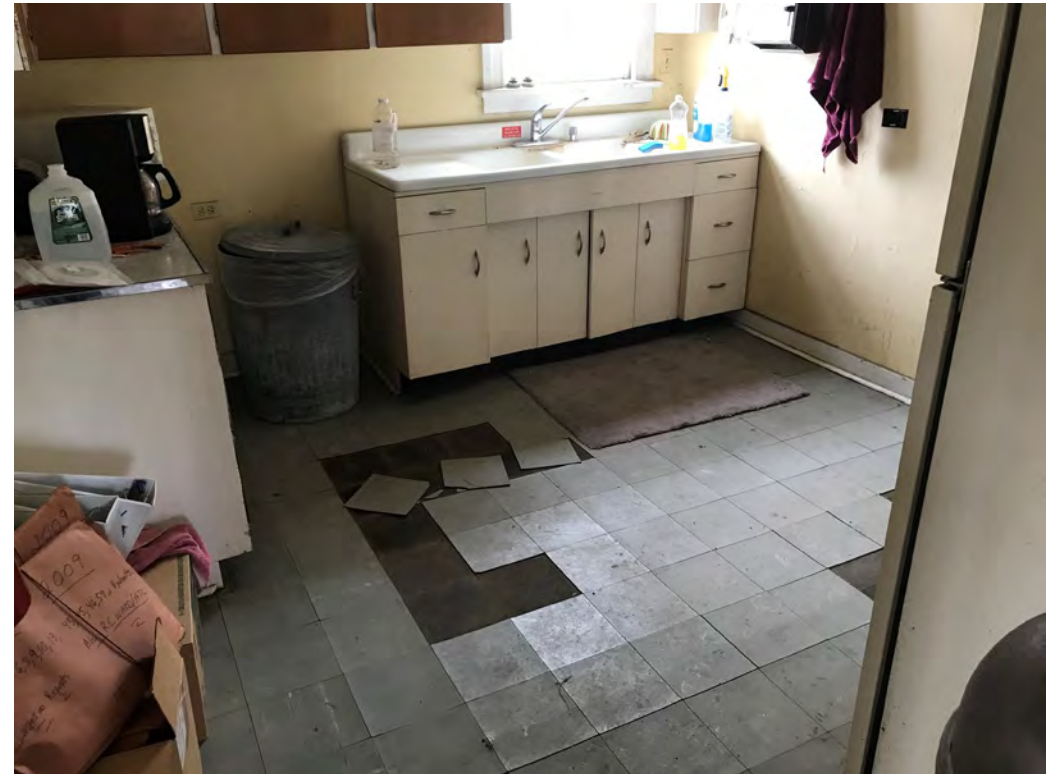
View of First Floor Kitchen looking Northeast
