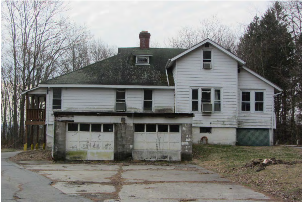
Photograph 1: Building 16 facing southeast to northwest elevation.
