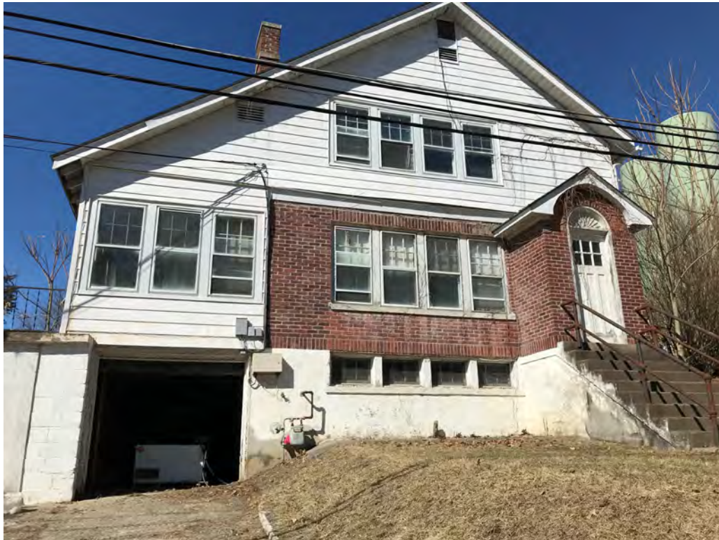
Exterior East Elevation
