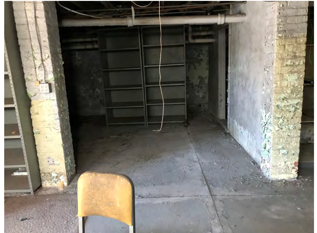
View of Basement looking West
