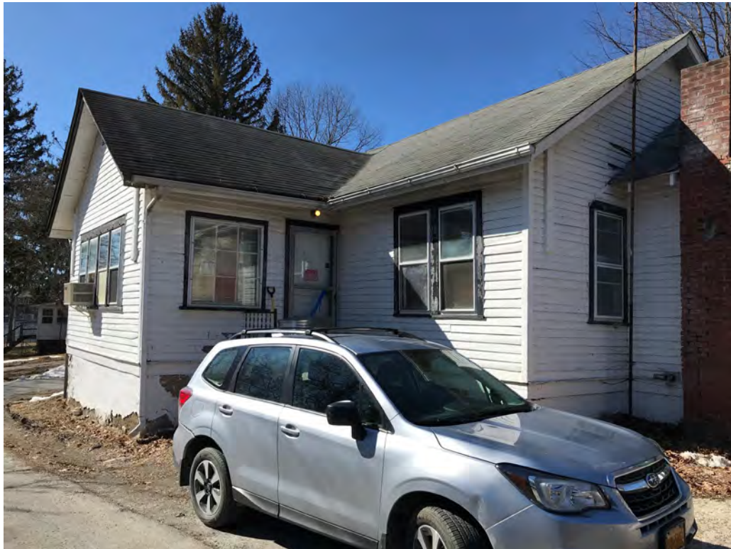
Exterior East Elevation
