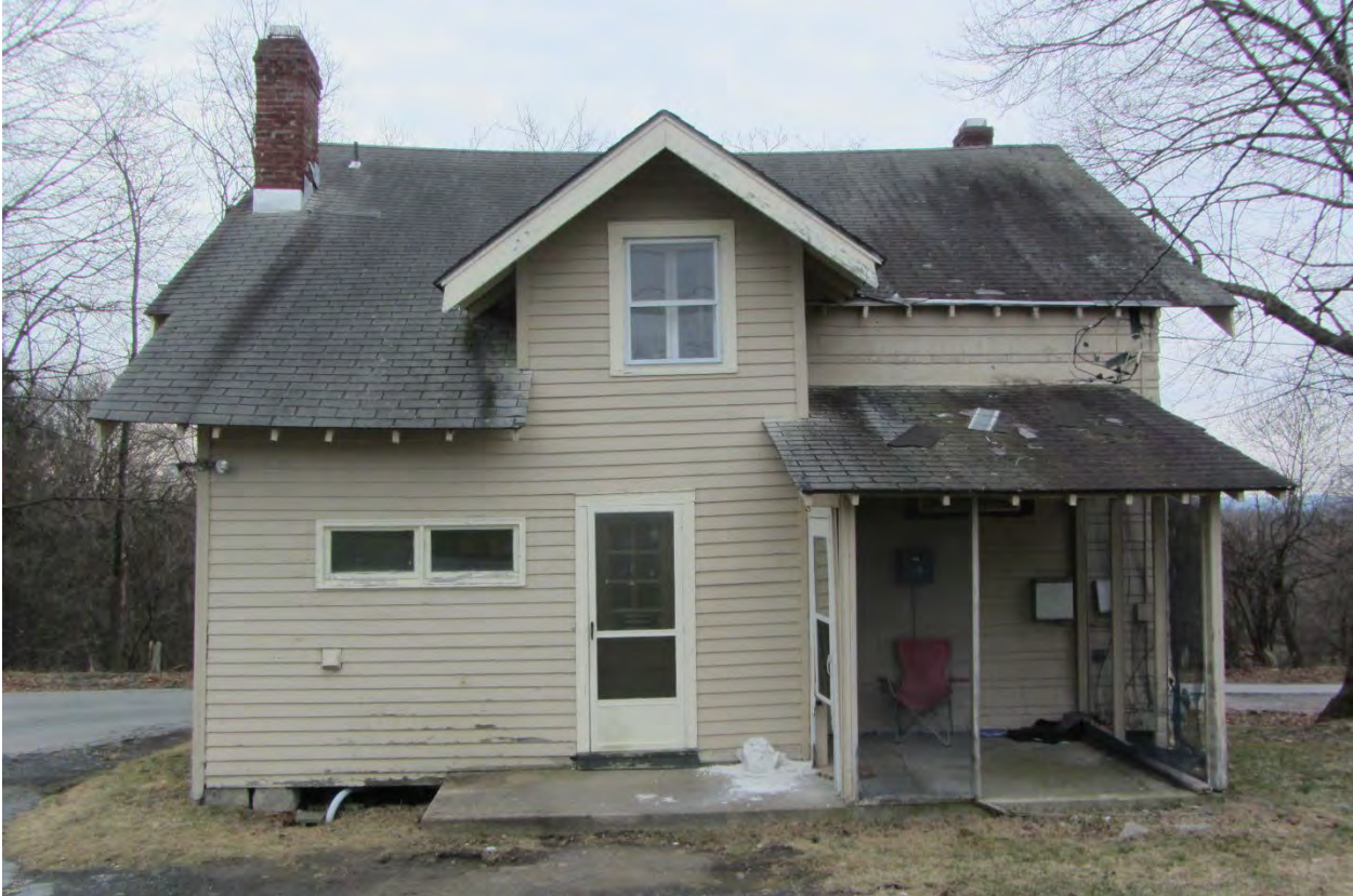
Photograph 8: Building 19 facing east to west elevation.
