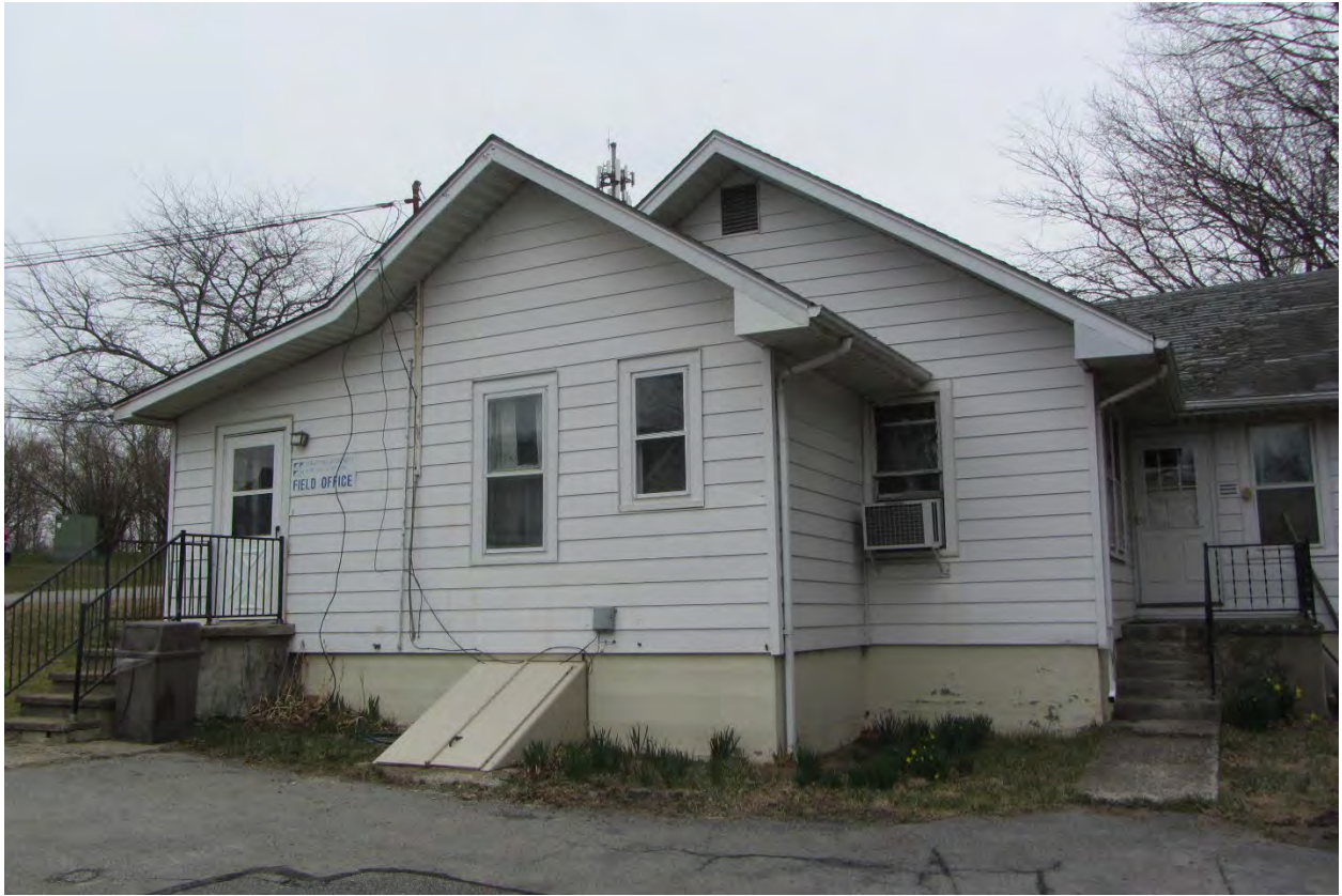
Photograph 5: Building 18 facing northeast to southwest elevation.
