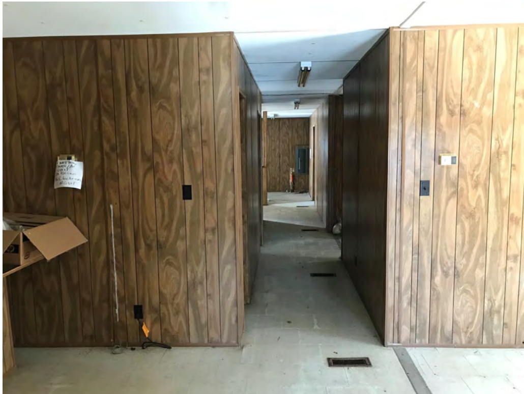
Interior South Conference Room with Mercury Ampoule Thermostats
