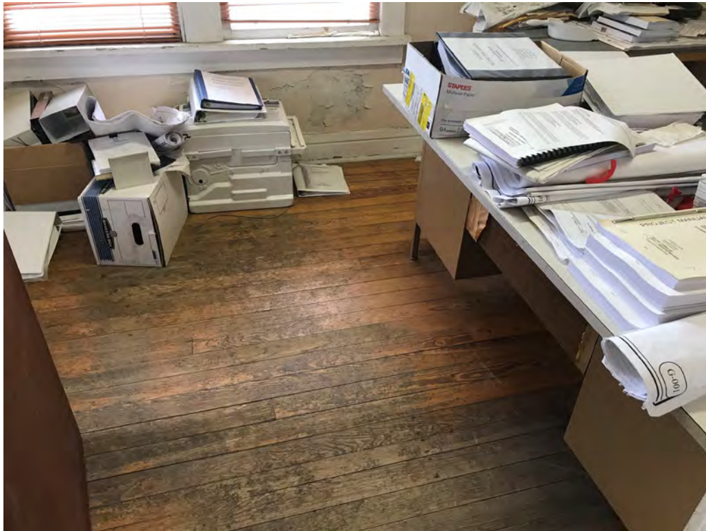
View of First Floor Northeast Office looking East
