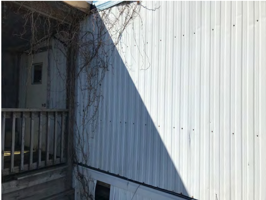
Exterior Northeast Elevation - Entrance
