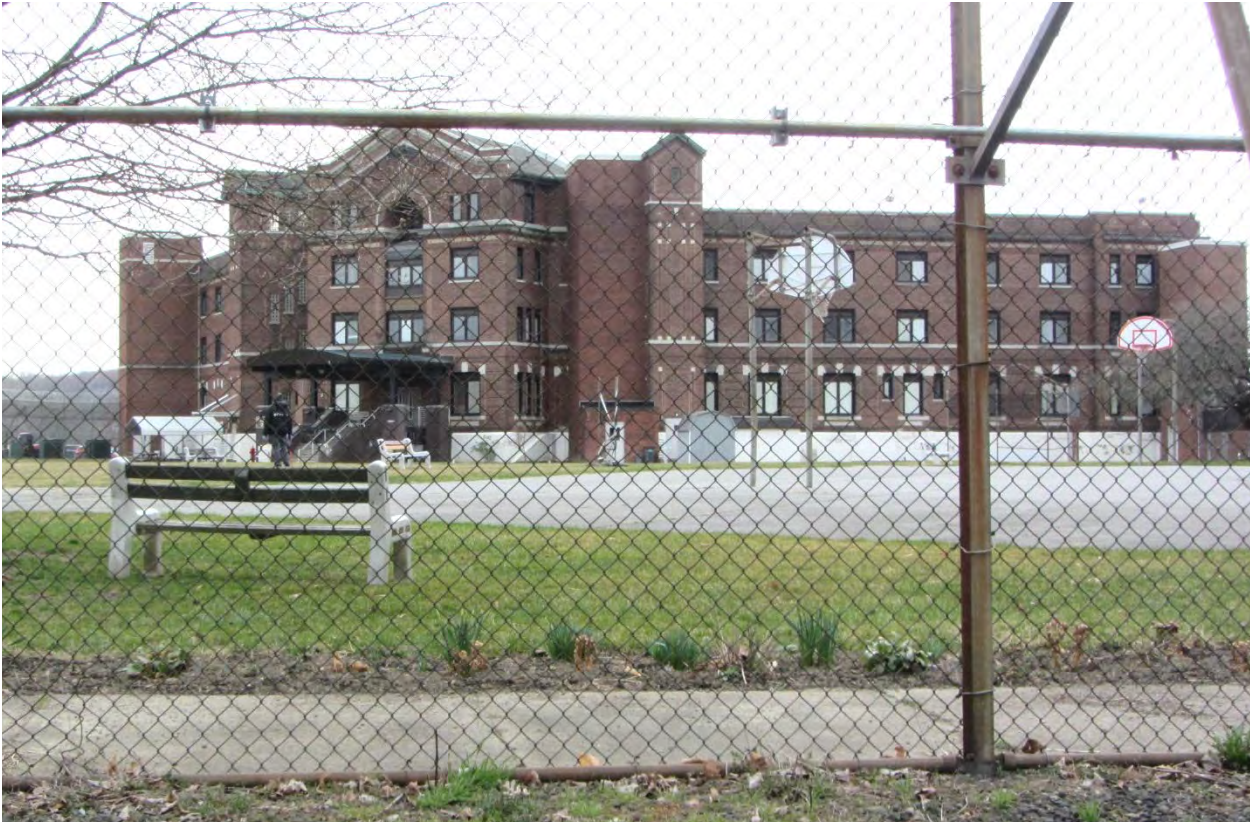
Photograph 20: Building No. 2 in existing complex facing southeast.
