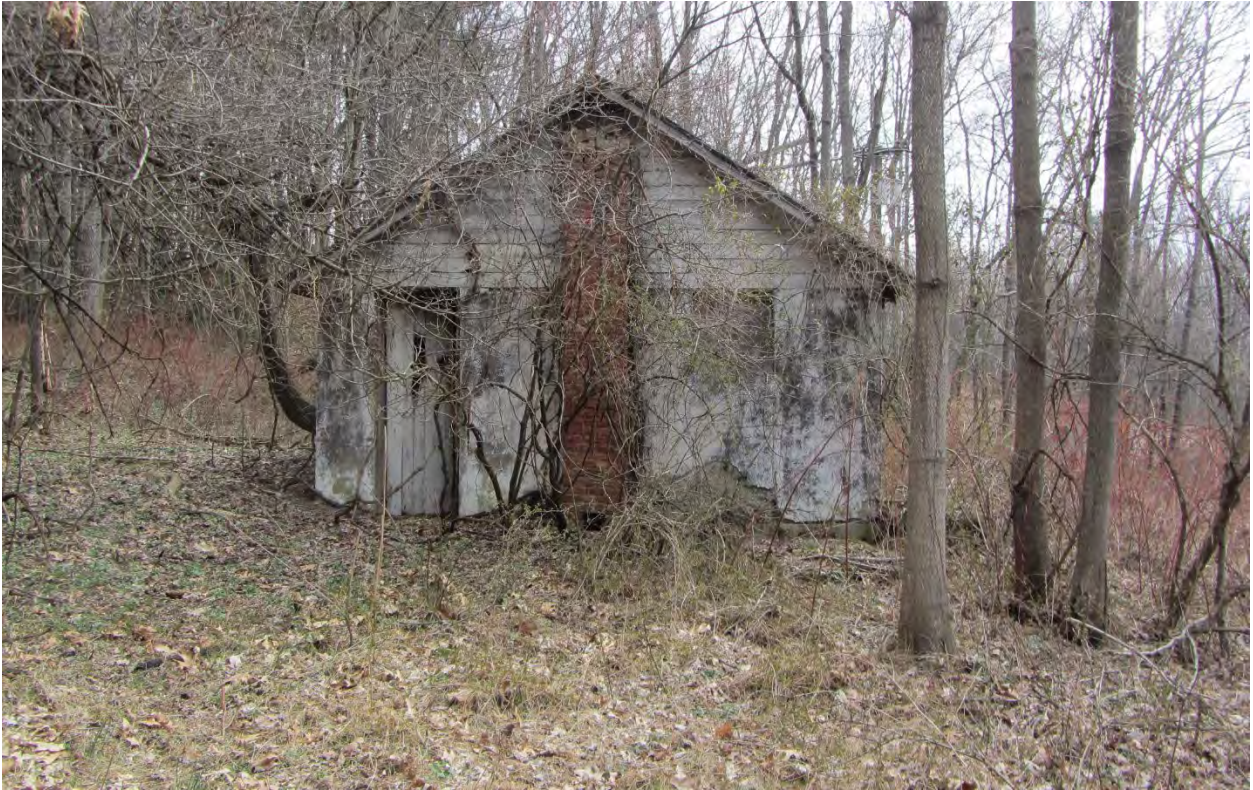
Photograph 25: Pump house north of the soccer field in northeastern corner of the project site, facing north.
