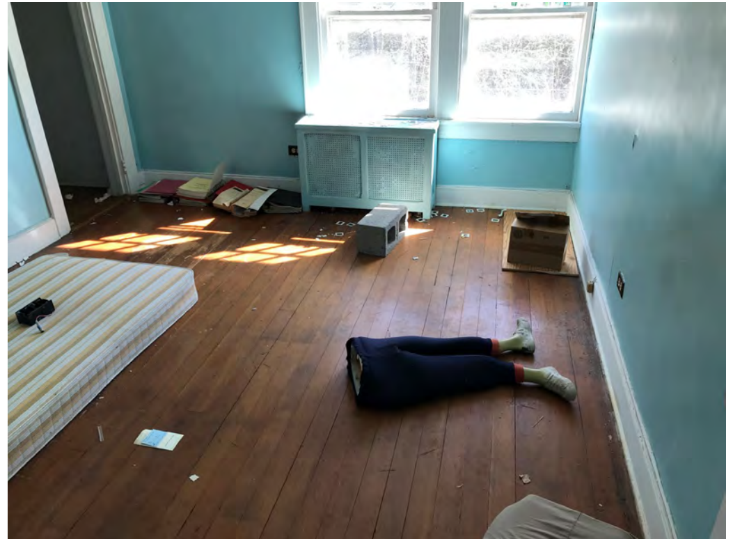
View of Second Floor MidEast Room looking East
