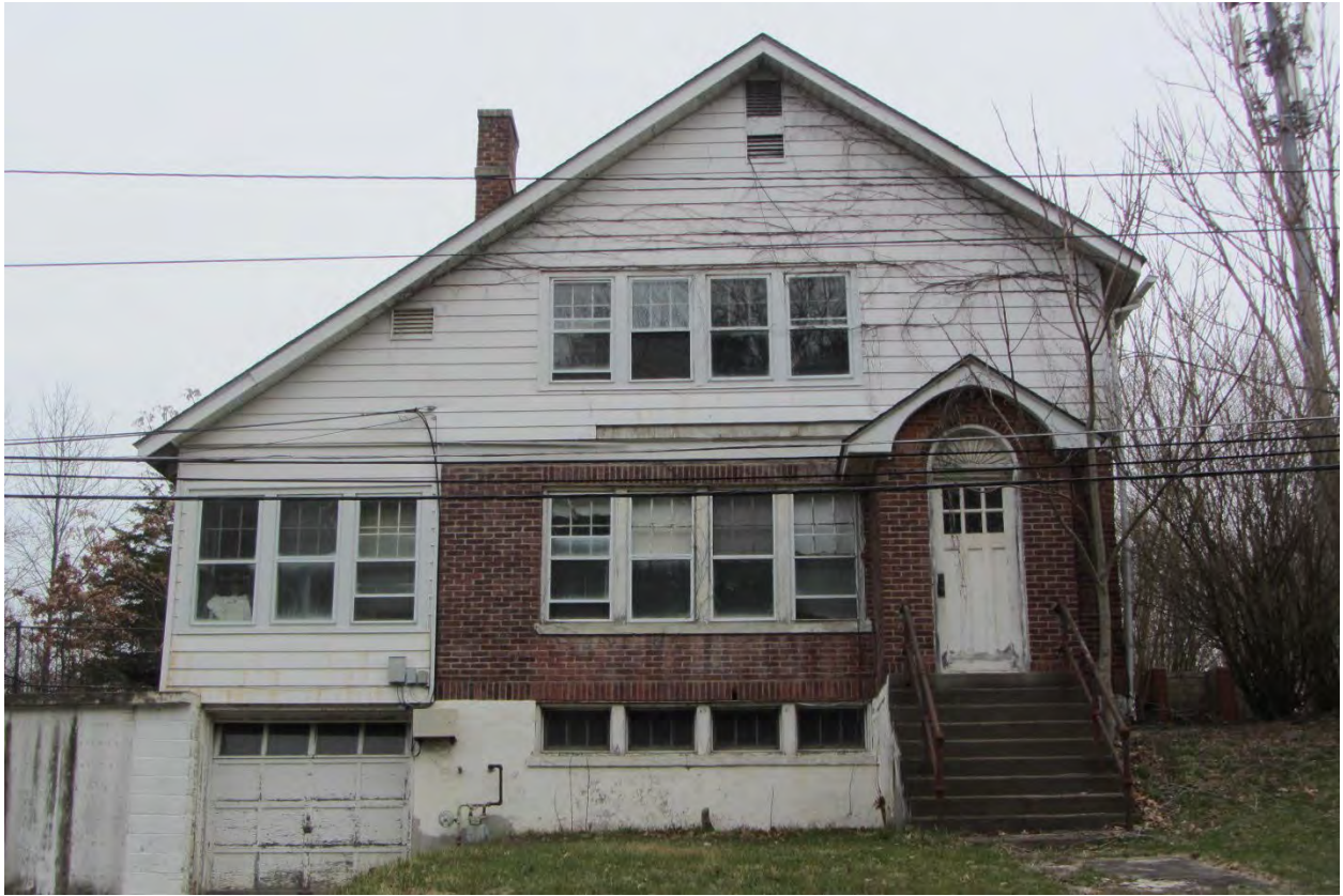
Photograph 3: Building 17 facing northwest to southeast elevation.
