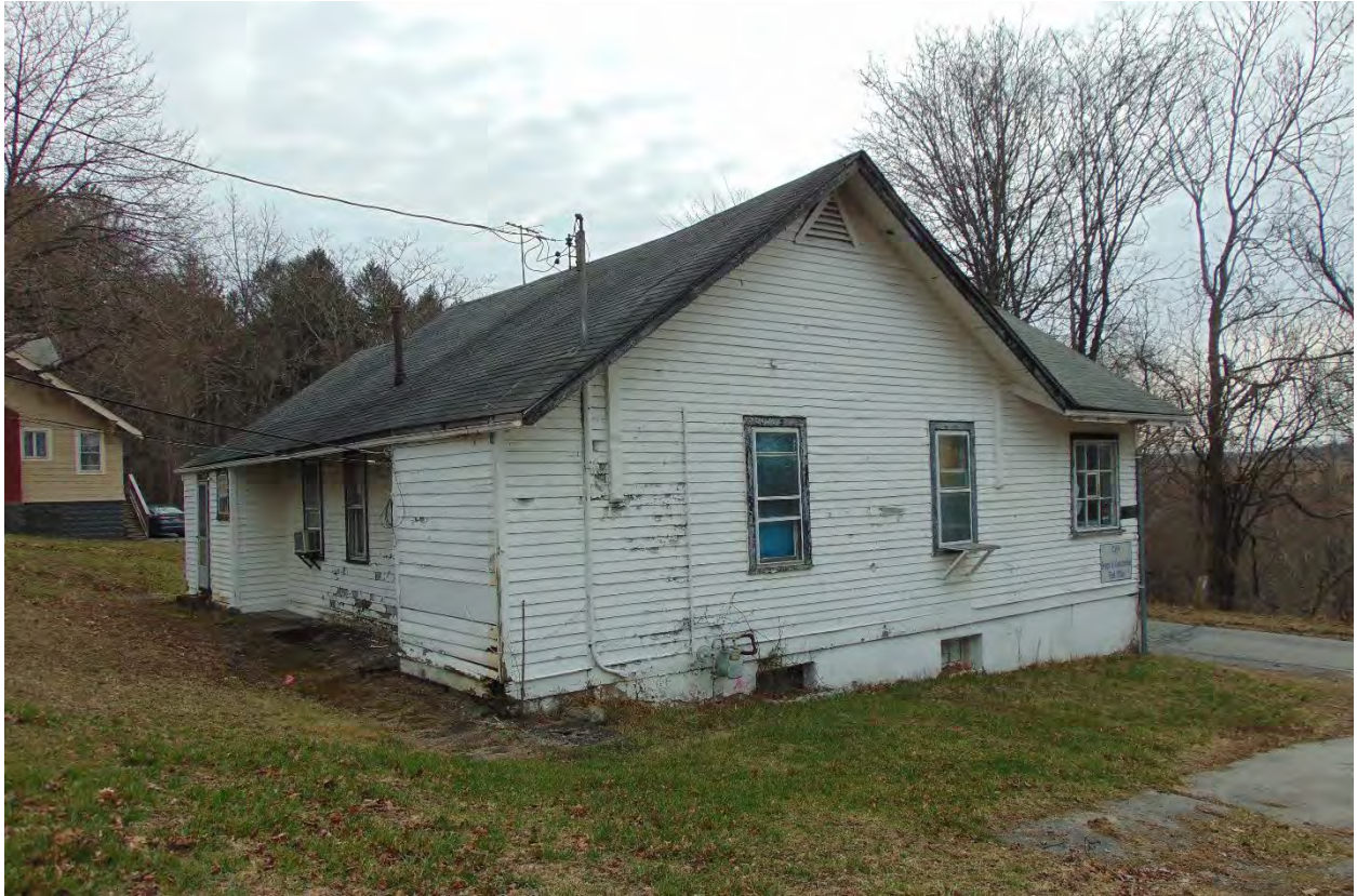
Photograph 9: Building 20 facing northeast to southwest elevation.
