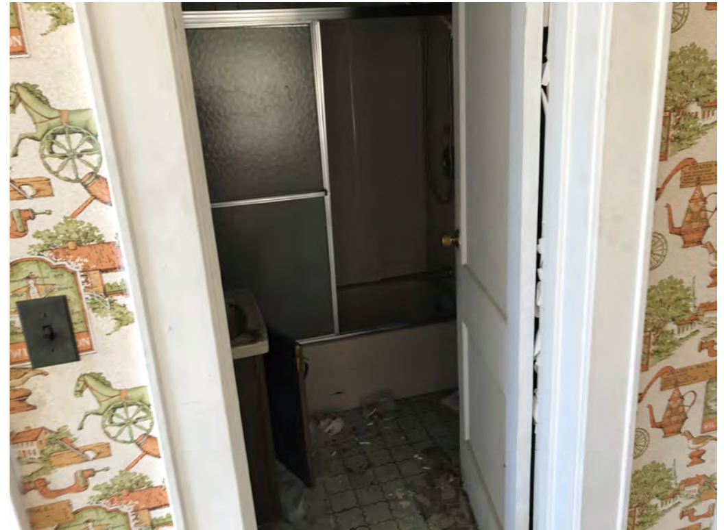
View of First Floor South Porch Bathroom looking West
