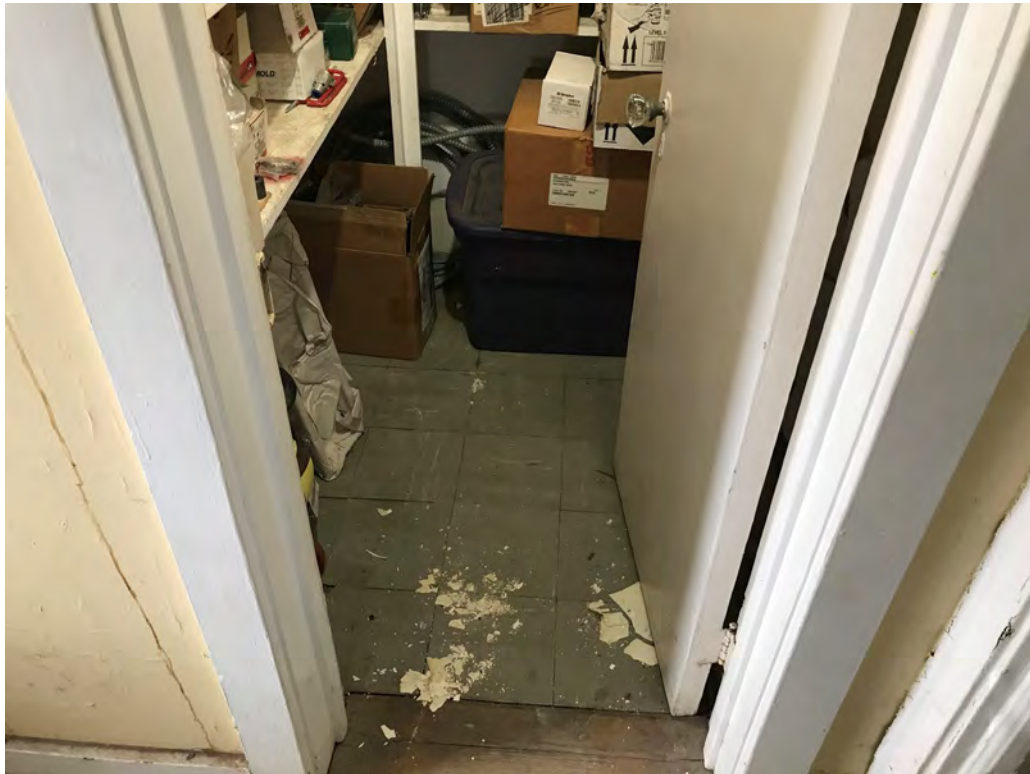
View of First Floor Pantry looking East
