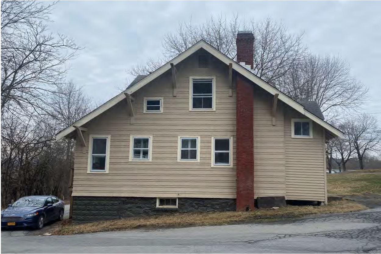
Photograph 7: Building 19 facing south to north elevation.
