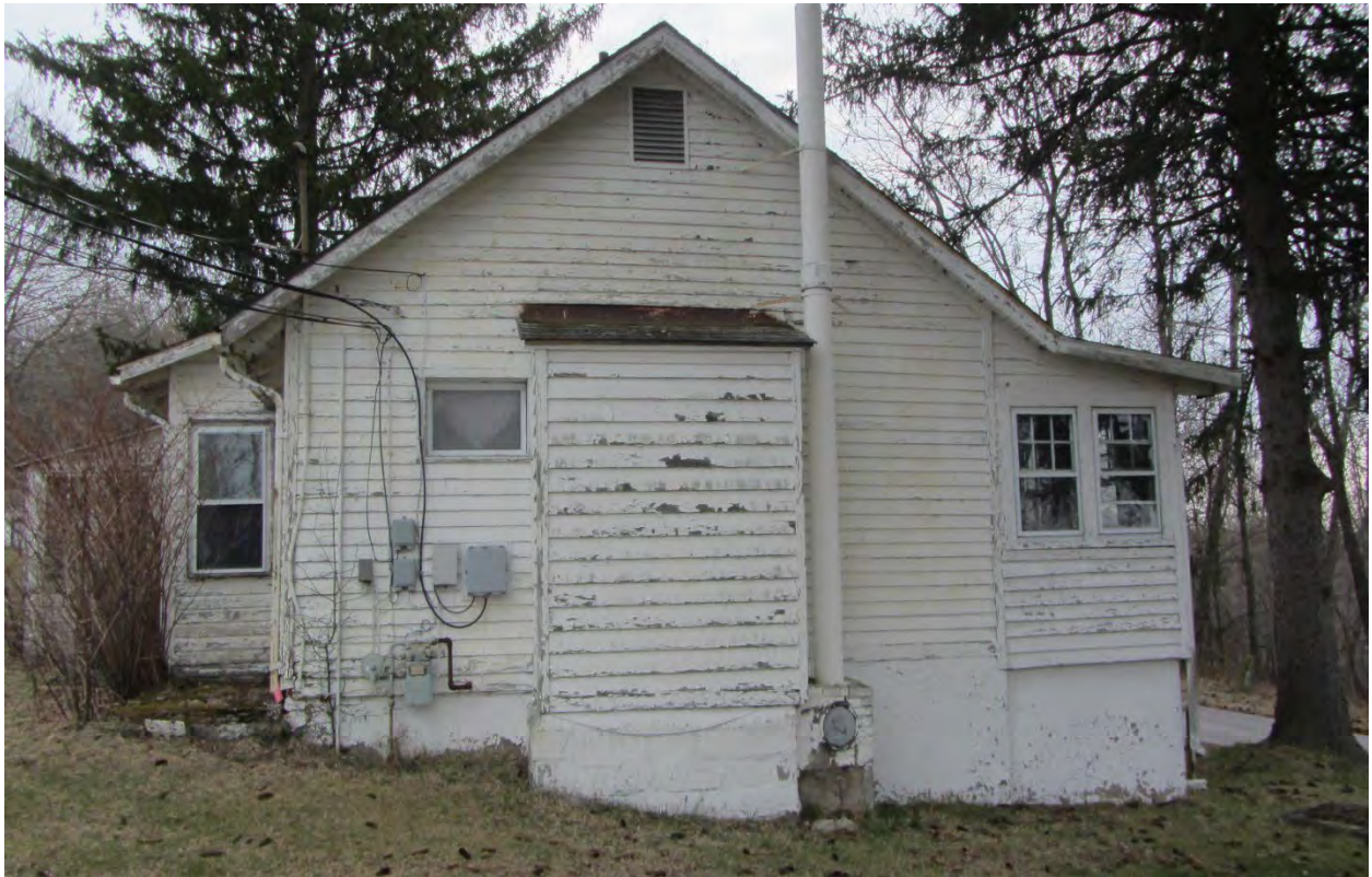
Photograph 12: Building 21 facing east to west elevation.
