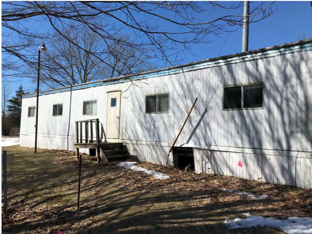
Exterior East Elevation
