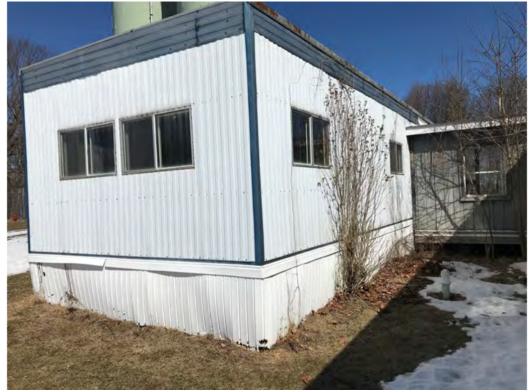
Exterior Southeast & South Elevation
