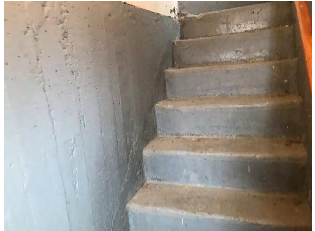
View of Basement Stair to First Floor looking West
