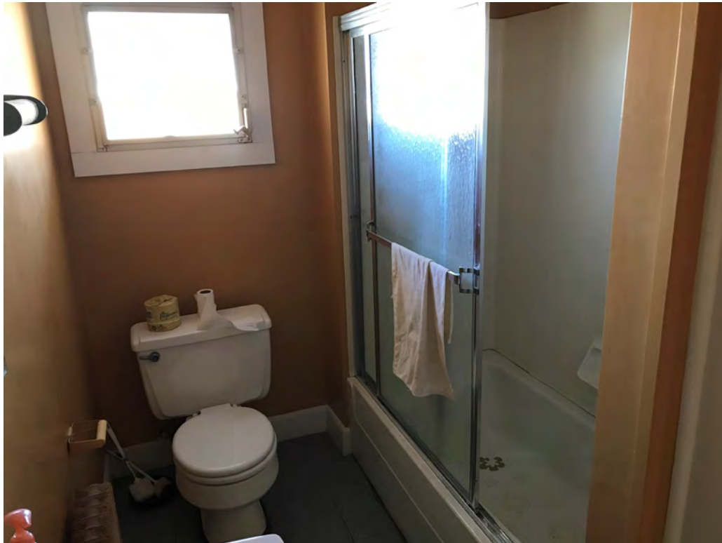
View of First Floor South Bathroom looking West
