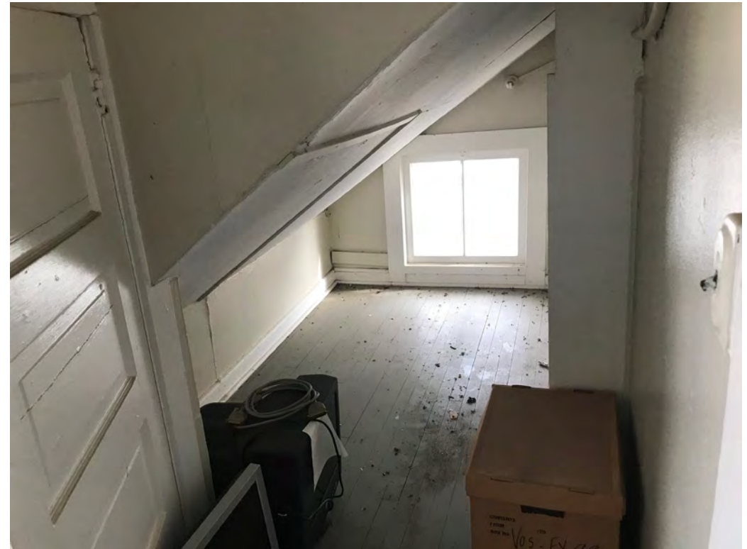
View of Second Floor Northwest Room looking North
