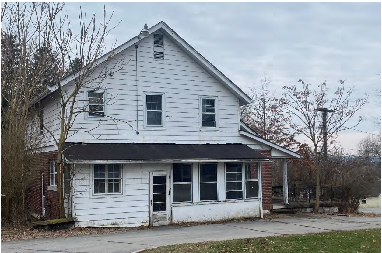
Photograph 4: Building 17 facing southeast to northwest elevation.
