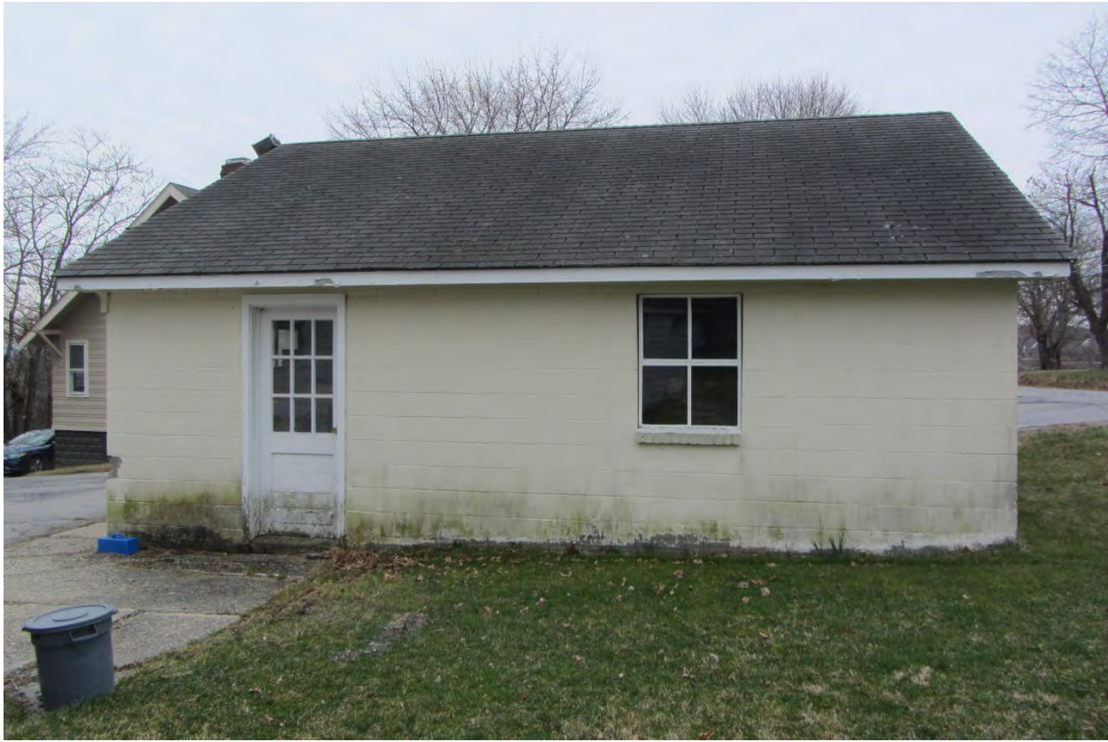
Photograph 14: Building 22 facing south to north and west elevations.
