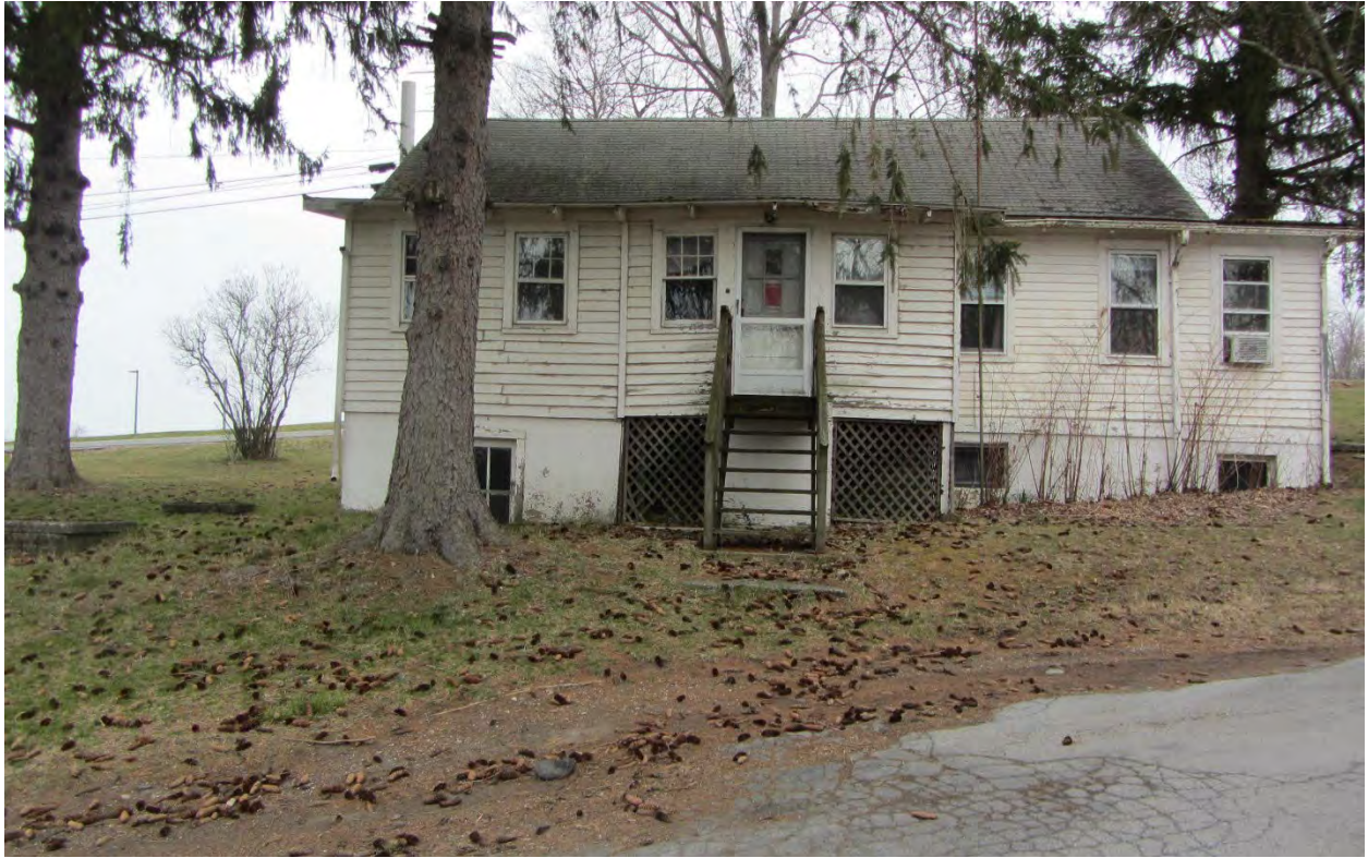
Photograph 11: Building 21 facing north to south elevation.
