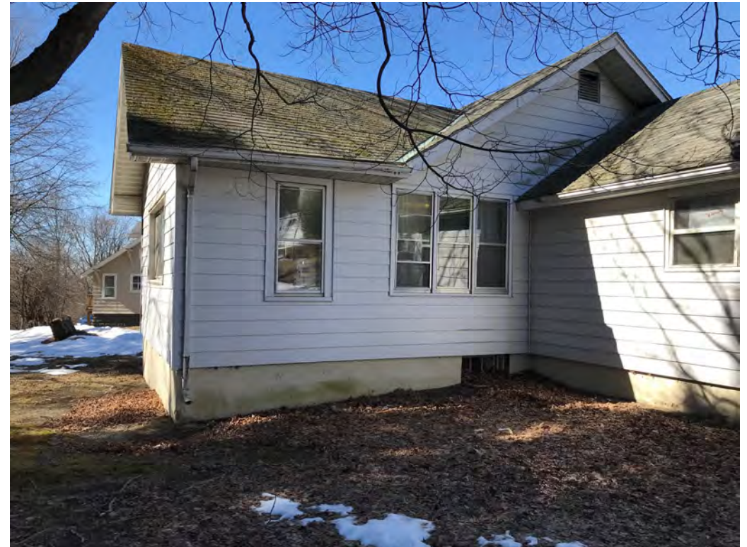
Exterior East Elevation
