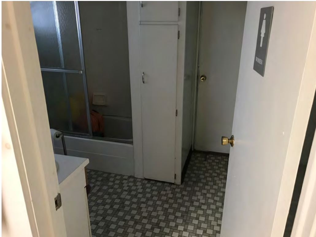
View of First Floor Southwest Bathroom looking West
