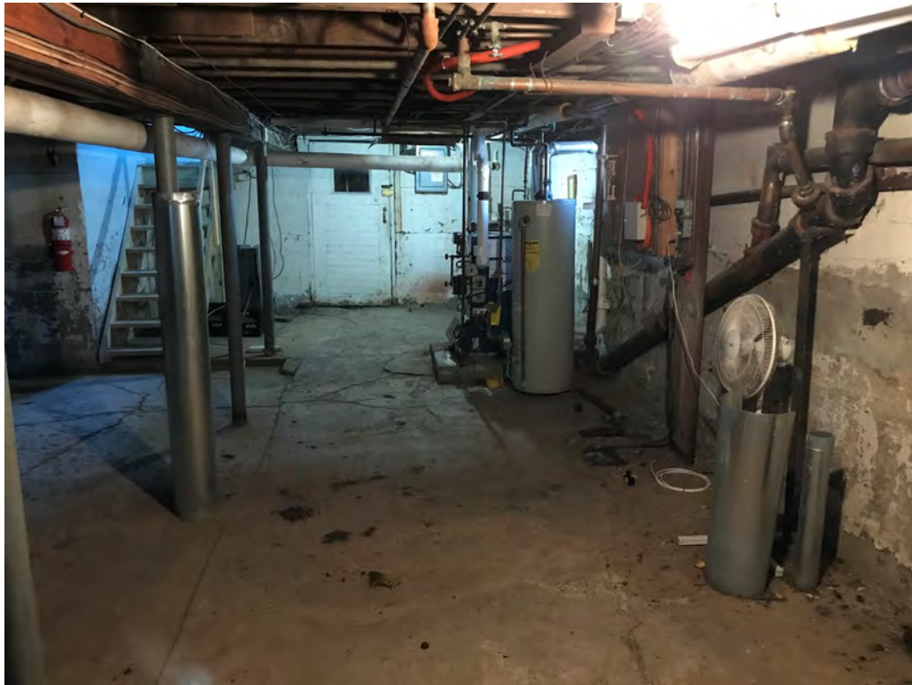
View of Basement looking South
