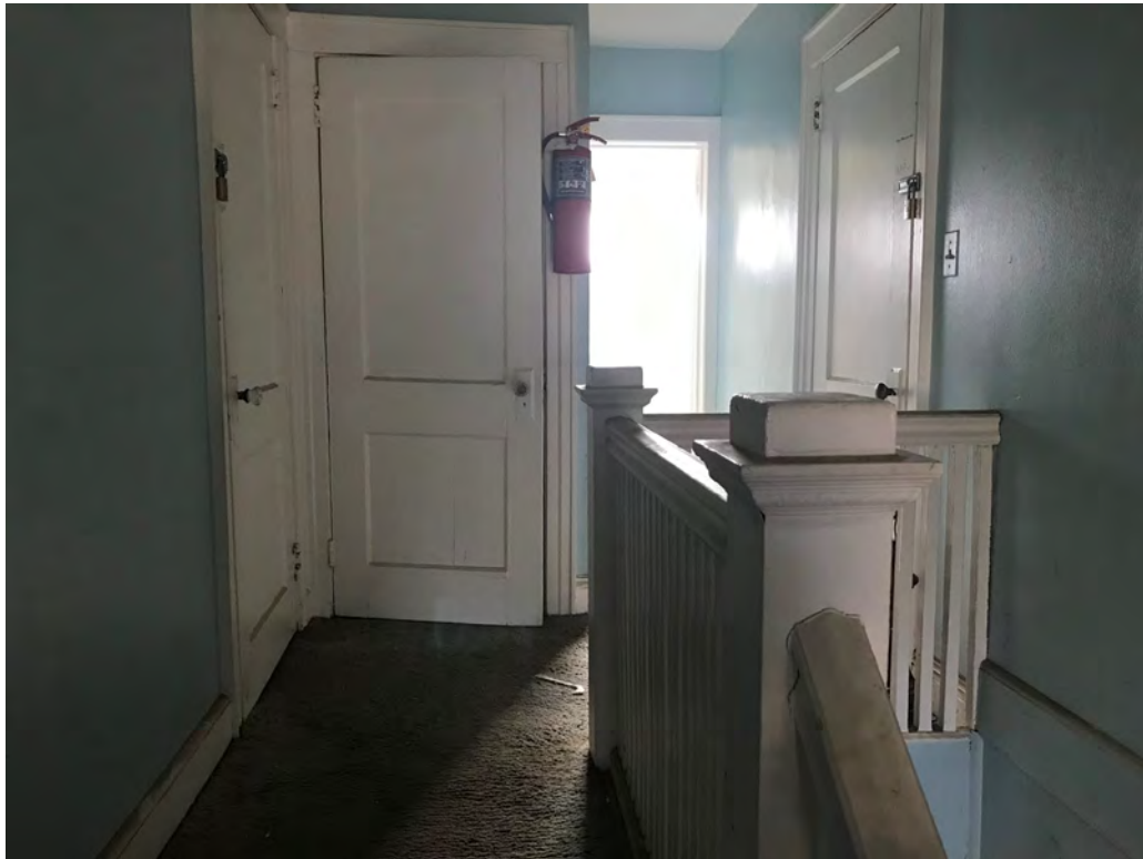
View of Second Floor Corridor looking East
