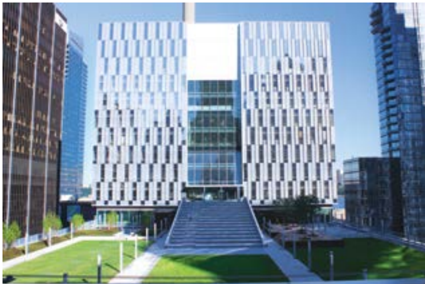
John Jay College of Criminal Justice: DASNY provided oversight of the design and construction of this new 625,000-square foot, multi-use building.
