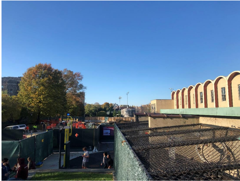
Photo 1: View of the Development Site and McGinley Campus Center Looking Northwest
