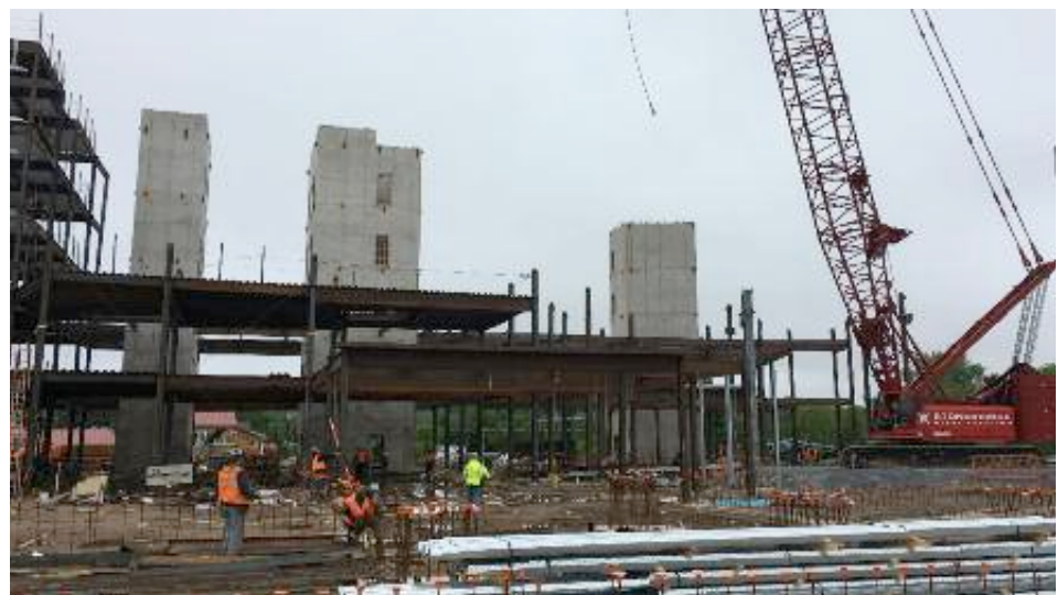
South Beach Psychiatric Center under construction
