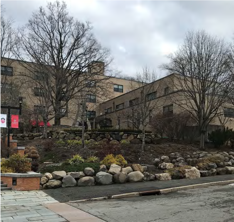
View of Existing St. Vincent Hall Rear Facade
