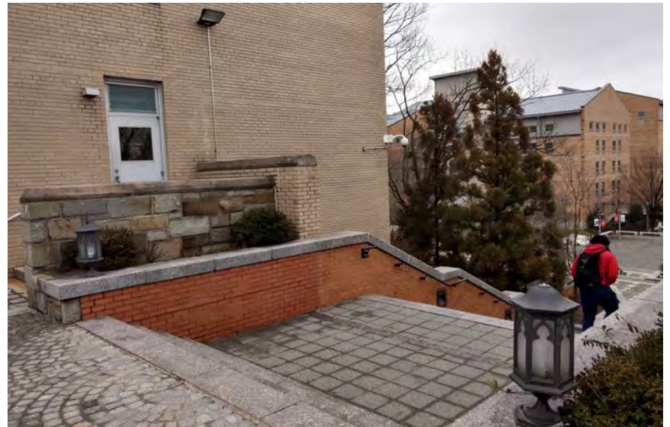
8 - Stairway Adjacent to St. Vincent Hall
