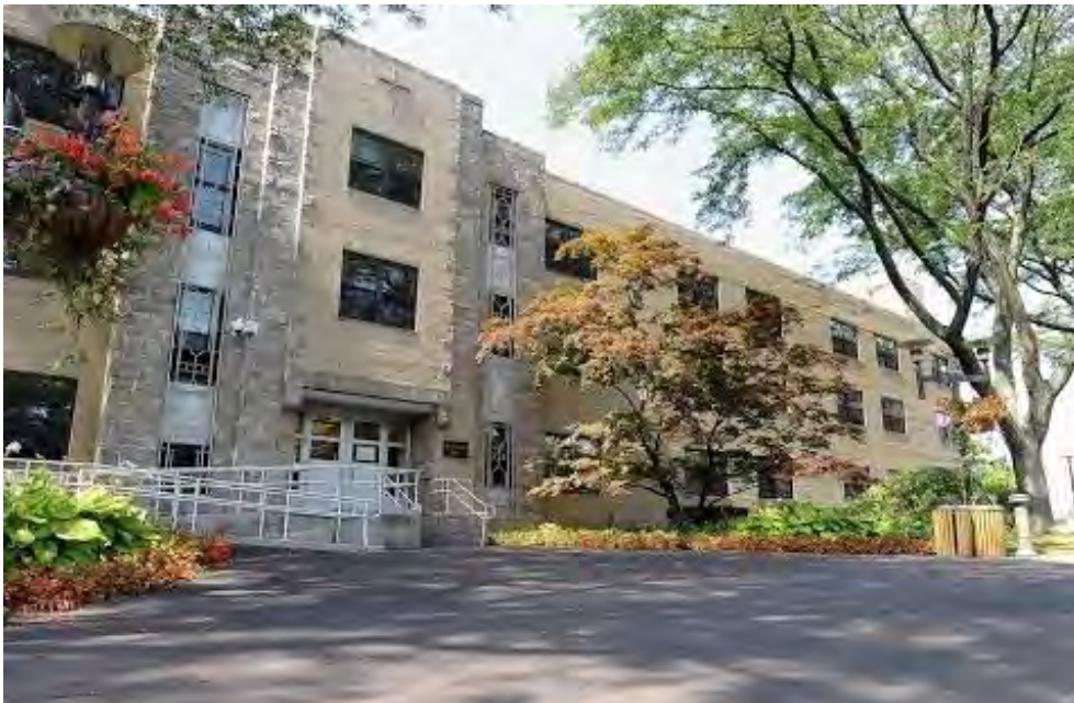
Image of the existing St. Vincent Hall Entry
