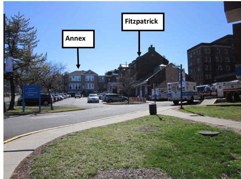
8. Fitzpatrick building and Annex
