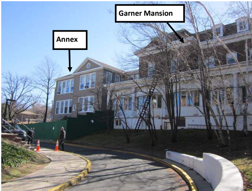
9. North side of Garner Mansion and Annex
