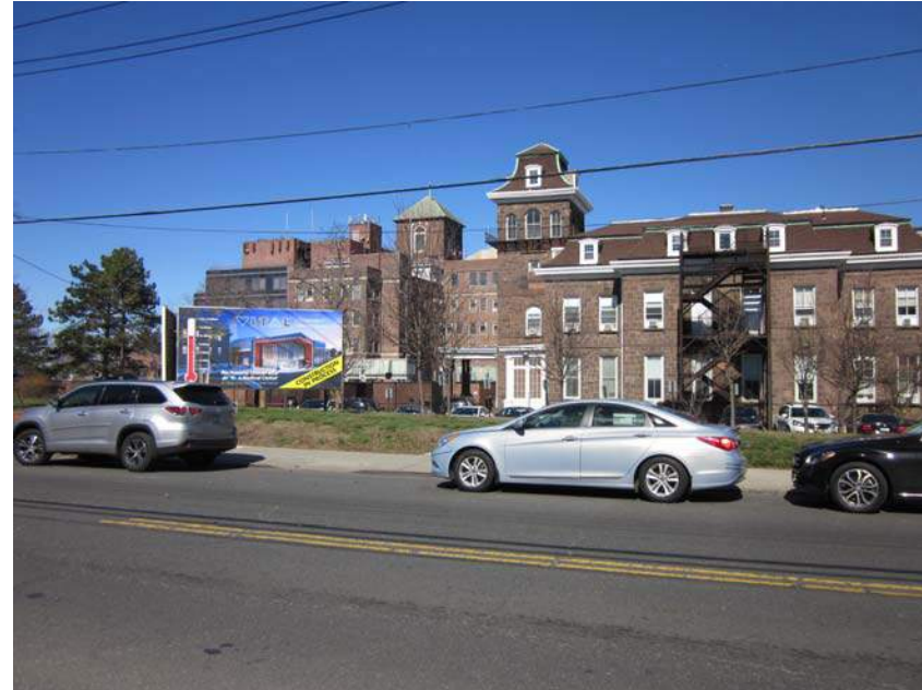
4. Looking north across Castleton Ave. toward project area
