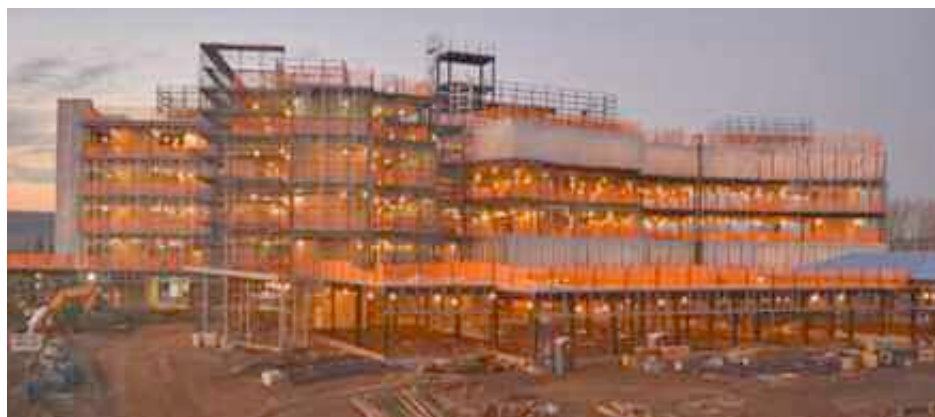
South Beach Psychiatric Center under construction.
