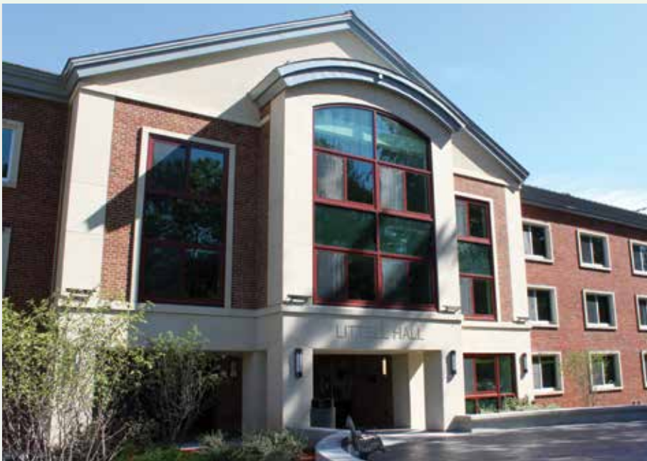
SUNY Oneonta Littell Hall —The 200-bed residence hall underwent an $8.5 million major renovation project, which included a new roof.
